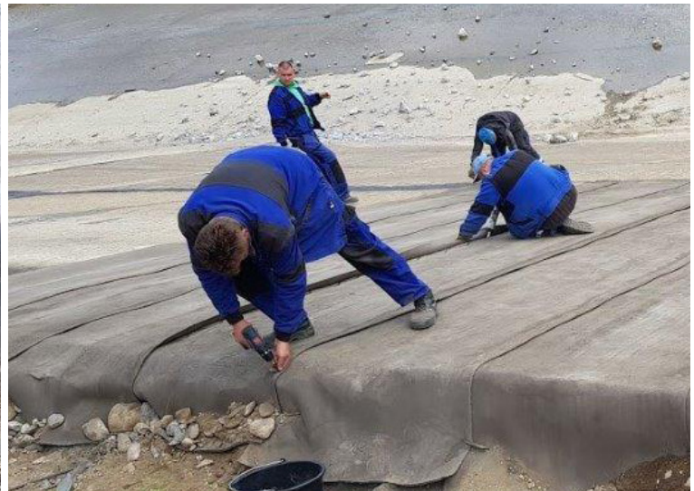
Overlapping layers joined with adhesive sealant and screws
