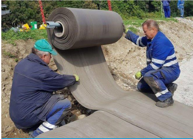
Deployment of the CC bulk rolls
