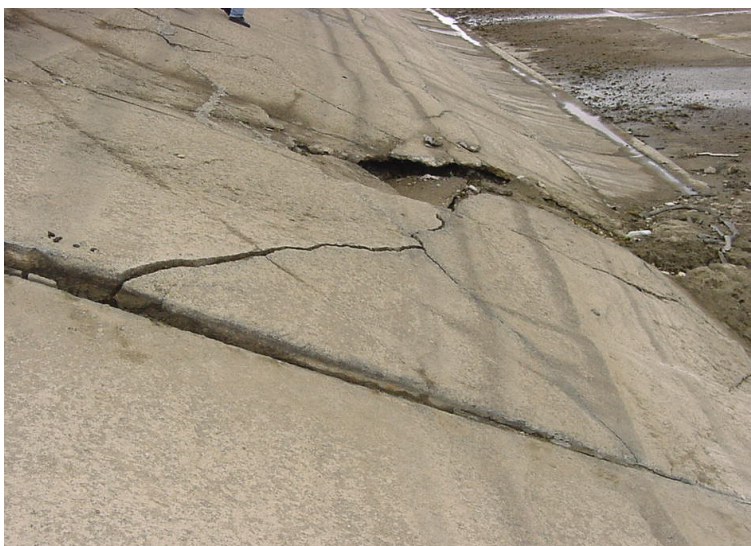
Large crack in section of concrete channel wall
