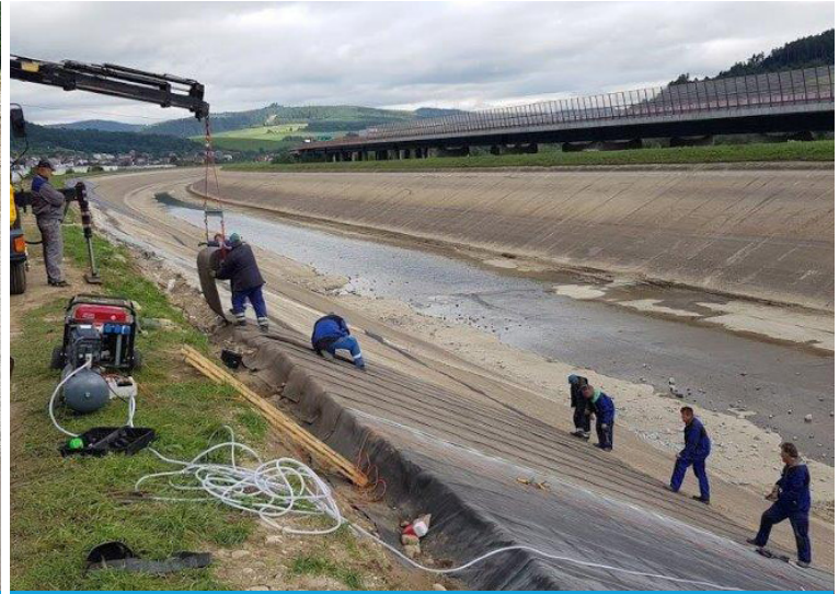
The CC was laid vertically down the slopes of the canal
