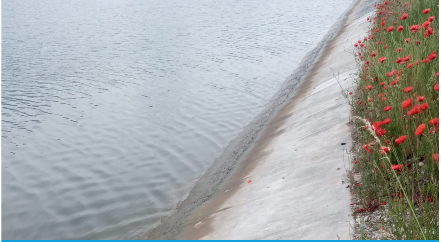
CC canal remediation installation revisited one year after completion
