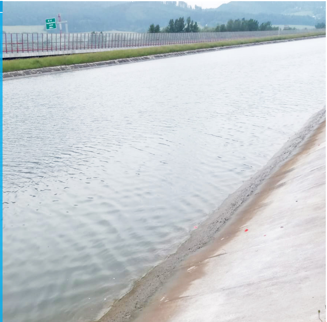
Completed CC concrete remediation installation in Slovakia
