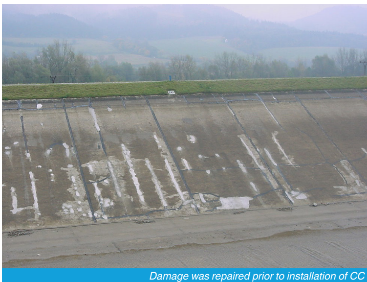
Large crack in section of concrete channel wall
