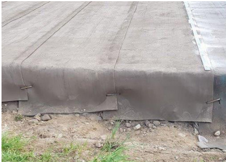
Ground pegs used to secure CC to ground
