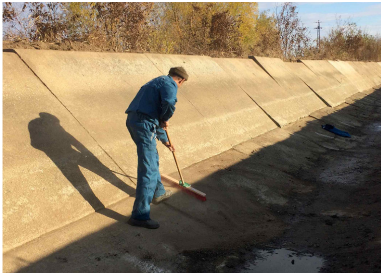
Removing dust and debris with sweeping brush
