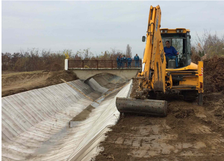
Backfilling anchor trenches
