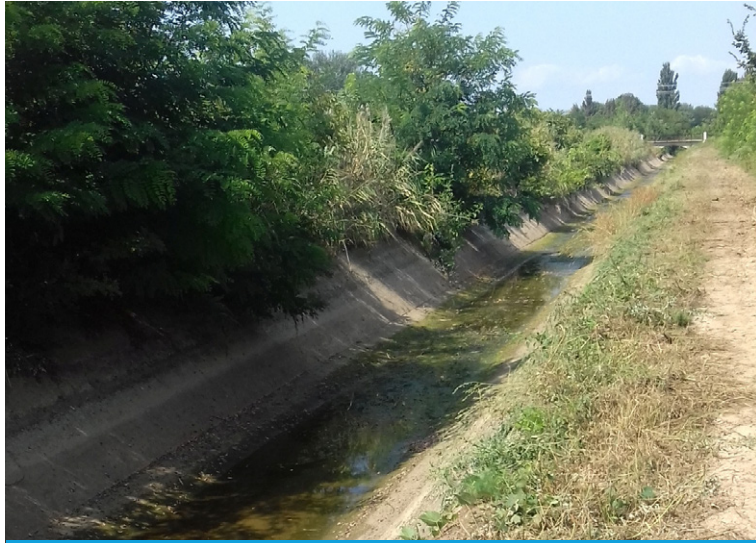
Canal prior to works
