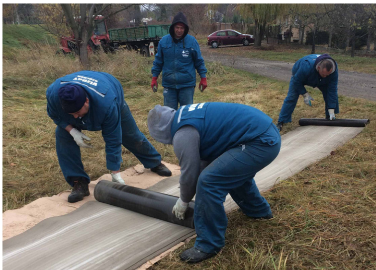
Batching CC for easier delivery to site
