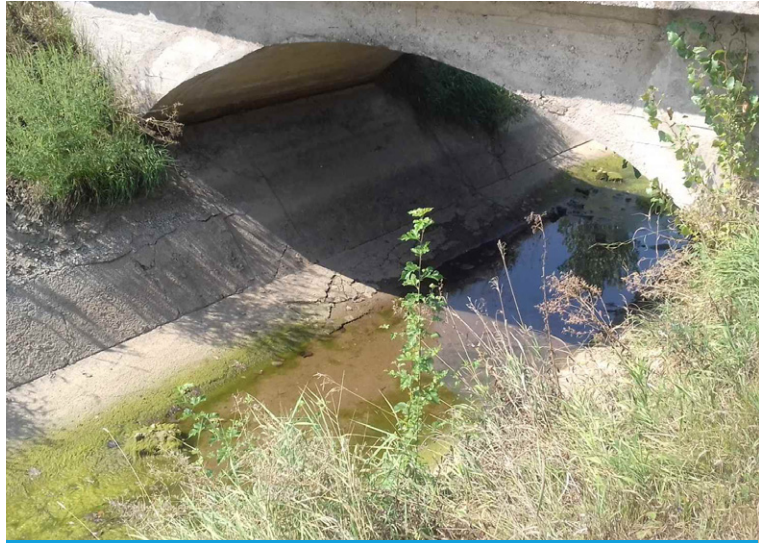
Section of canal below a bridge
