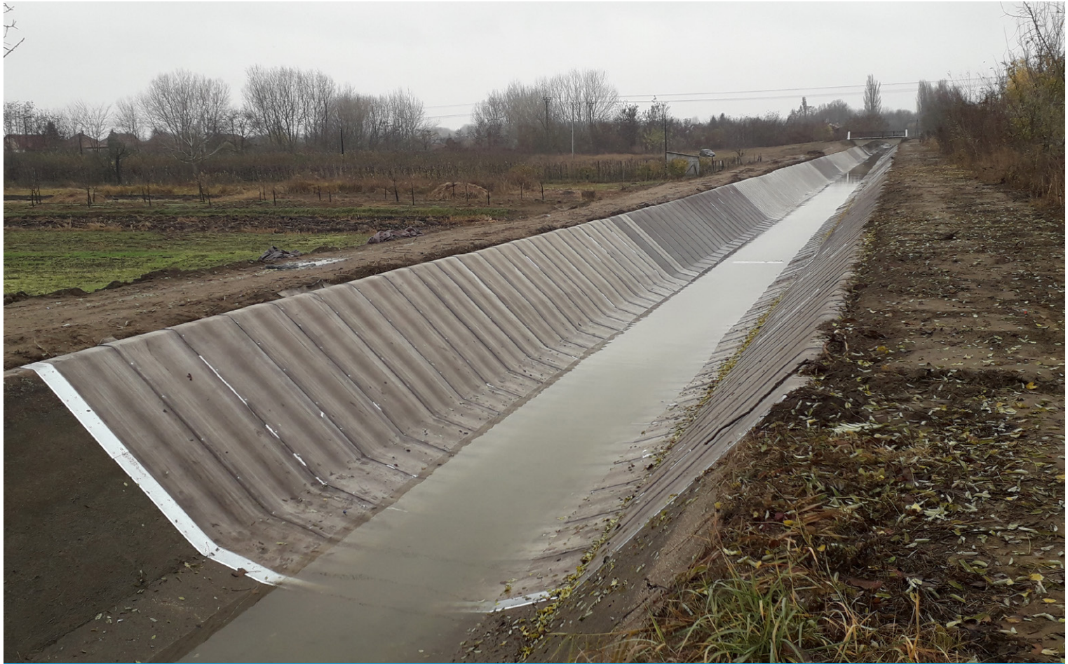
Completed remediation installation
