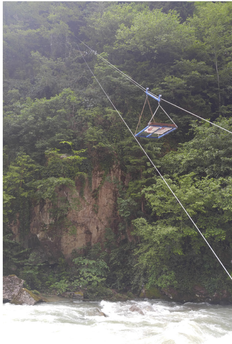
The batched rolls had to be winched to the site on a makeshift cable car
