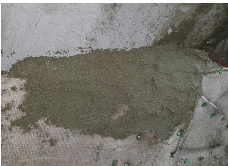
Mortar and sealant was used to prevent ingress at the edges of the CC
