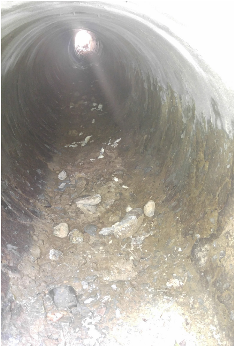
The inside of the pipe had to be cleared of rocks and debris prior to works
