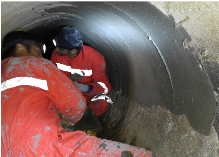
Repair works were carried out with mortar prior to installation
