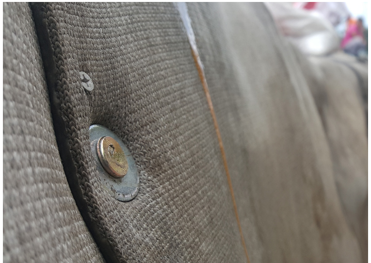
Anchor wedges were used to fix the CC to the channel walls
