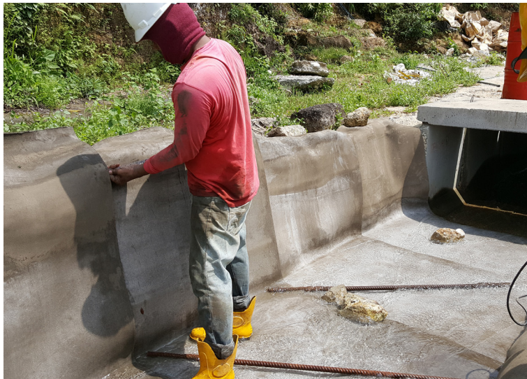
The CC was laid transversely in flowing water
