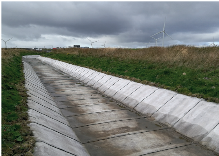
Anchor trenches backfilled on either side of channel
