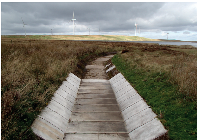
Localised damaged areas of the channel remediated with CC
