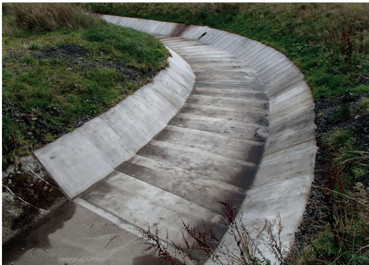
CC terminated into anchor trench and backfilled with concrete
