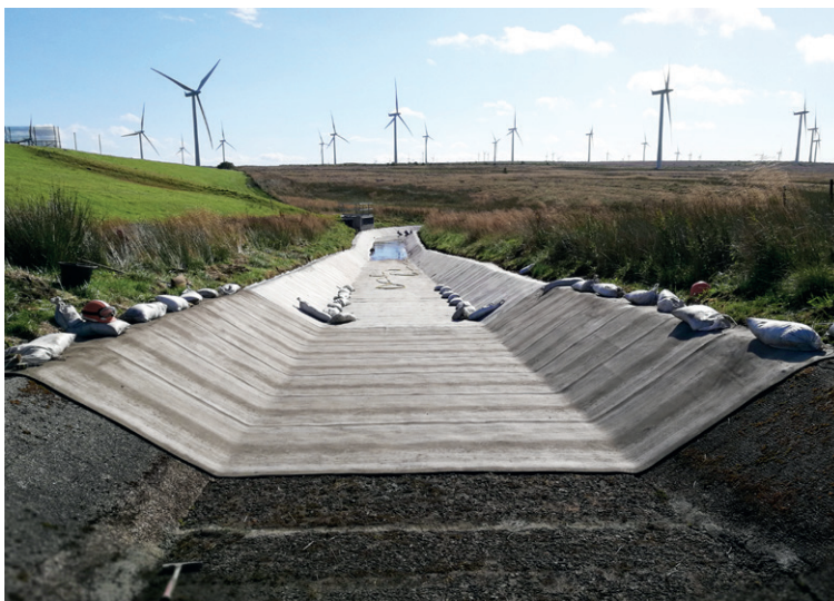
CC batched lengths laid transversely across the channel
