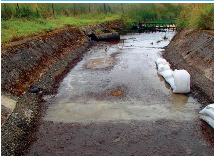
80mm perforated pipe installed to divert underlying water back into channel
