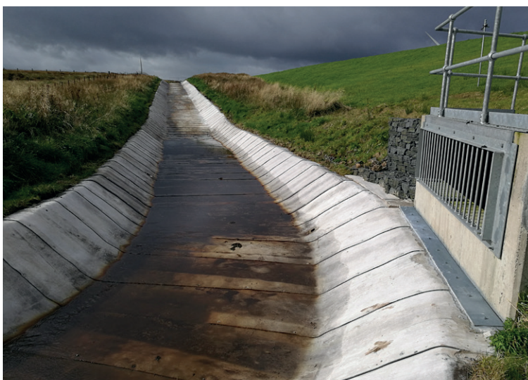
CC lined spillway channel with steel batten bar termination at siphon outlet
