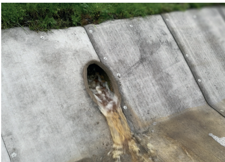
CC easily cut & grouted around pipe discharge points
