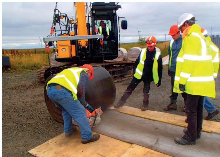
CC8 roll dispensed with spreader beam & cut to length off site
