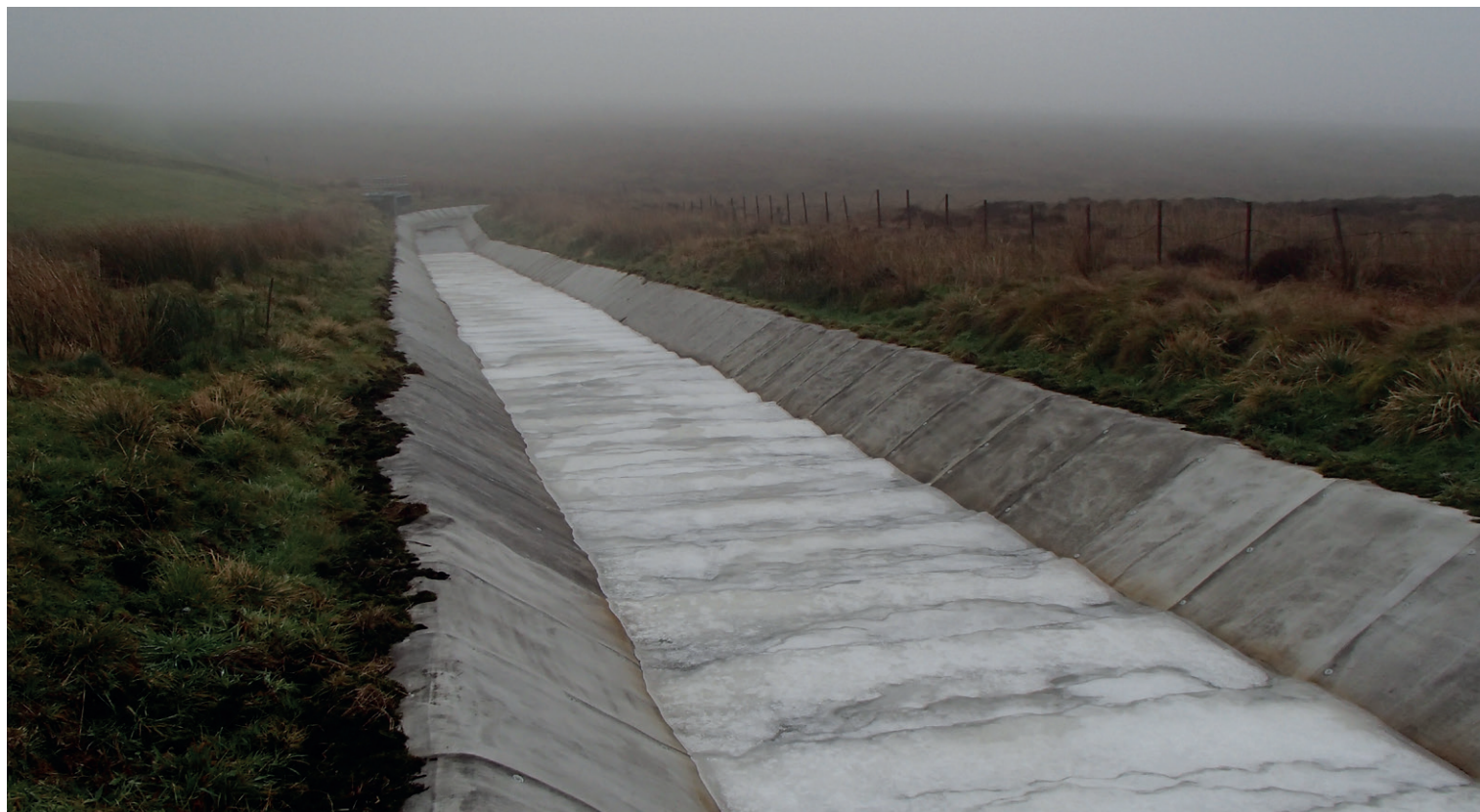
CC lined channel during winter period showing no signs of degradation
