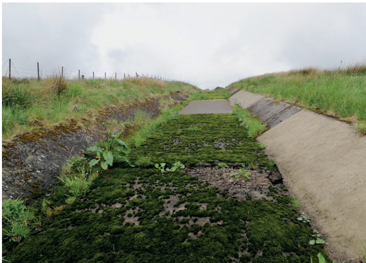
Algae & vegetation growth with existing concrete slabs damaged
