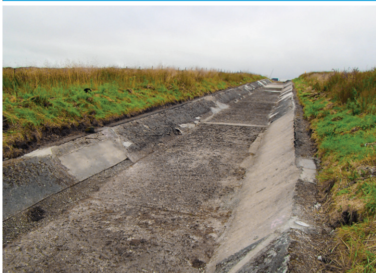
Vegetation removed & voids filled with flexible cementitious mortar
