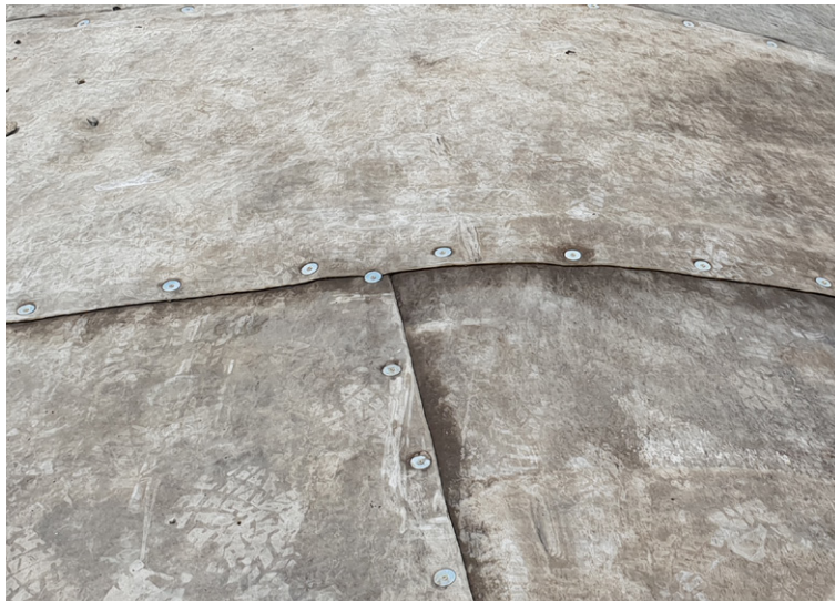
Stainless steel wedge anchors used to fix CC to concrete below
