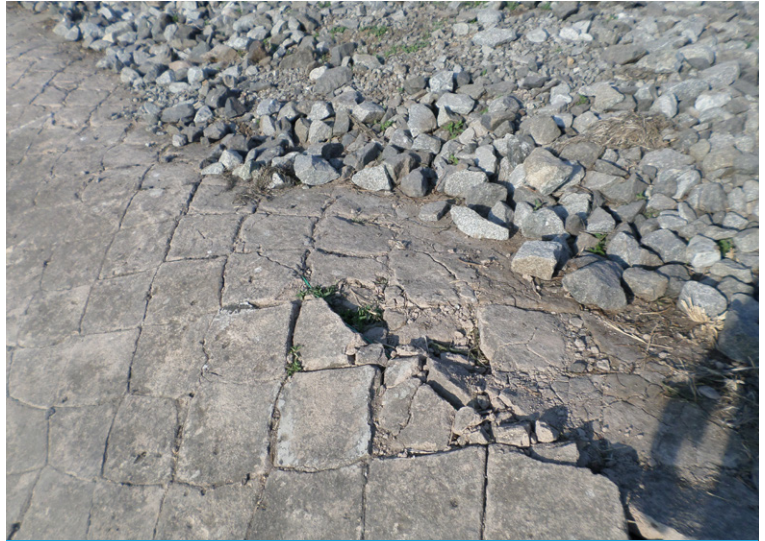
Significant cracking was found at a number of points around the dam
