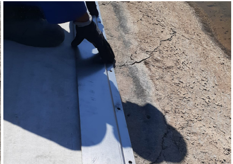
Stainless steel plate allowing expansion and contraction beneath
