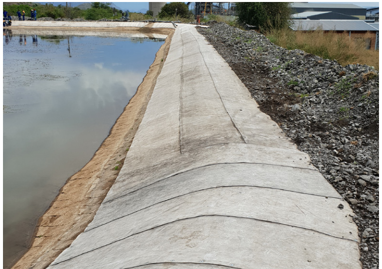
Transverse and vertical layups used to accommodate the shape of the dam
