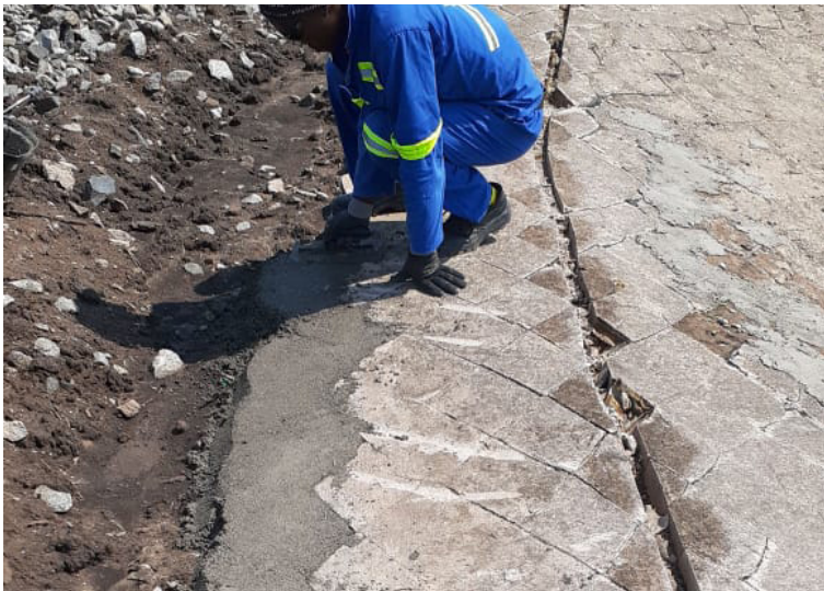
Large cracks were filled with cement-stabilised gravel
