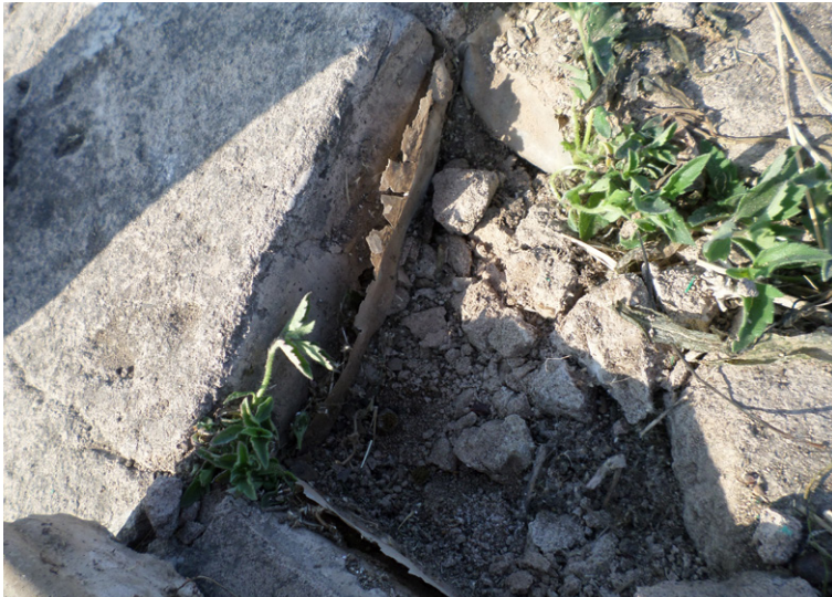
Geocell section showing significant damage where concrete has broken up
