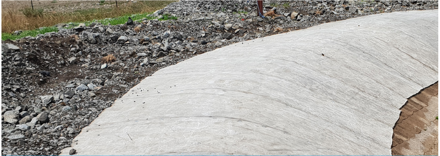
Upper edge of CC lengths captured in anchor trench
