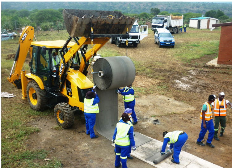
CC bulk rolls dispensed and cut to length on site
