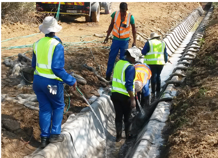
Hydration and compression of joints
