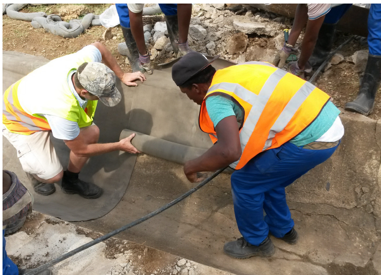
CC was laid transversely across canal width
