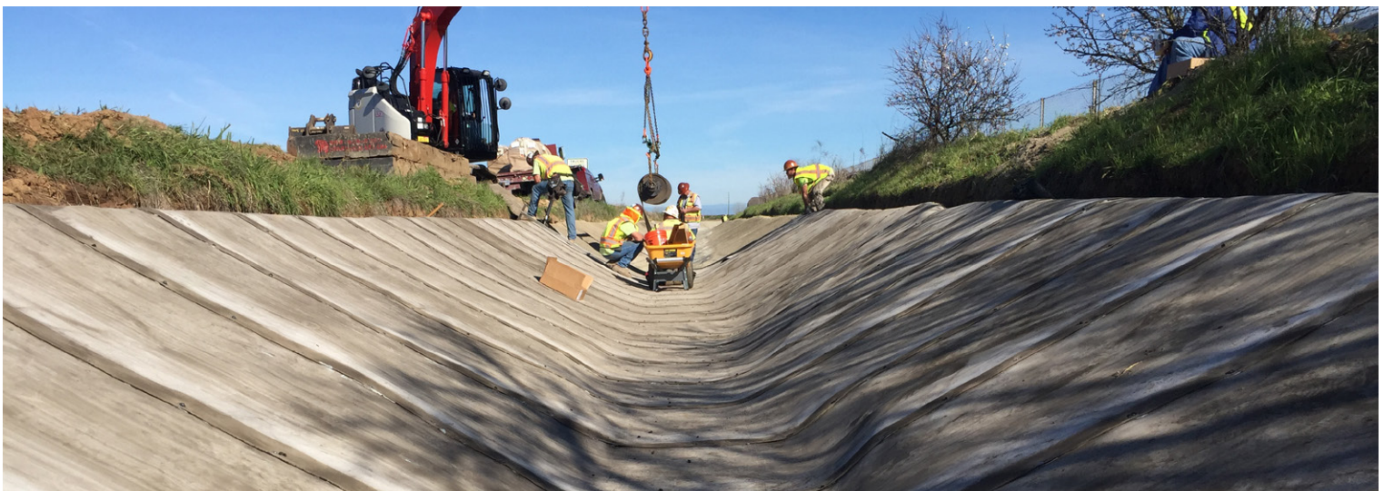
Deployment of CC bulk roll
