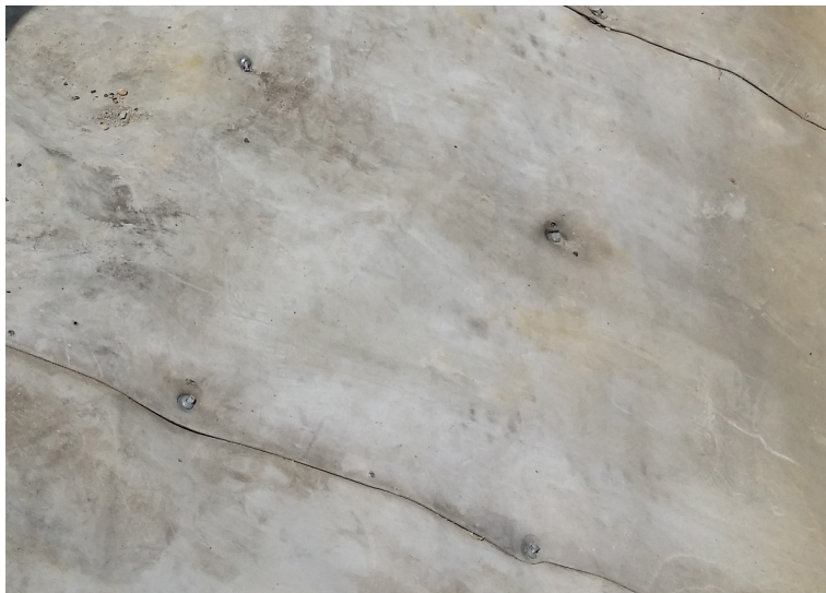
Screws were used to joint overlapping layers of CC
