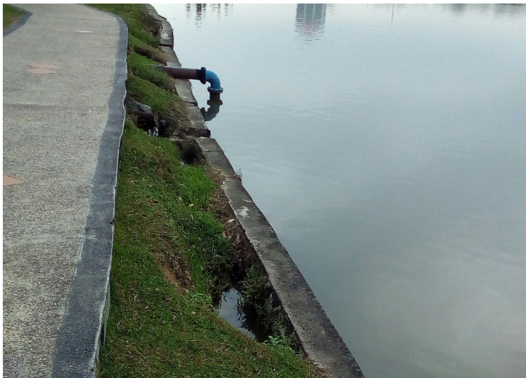
Voids created by erosion behind retaining walls
