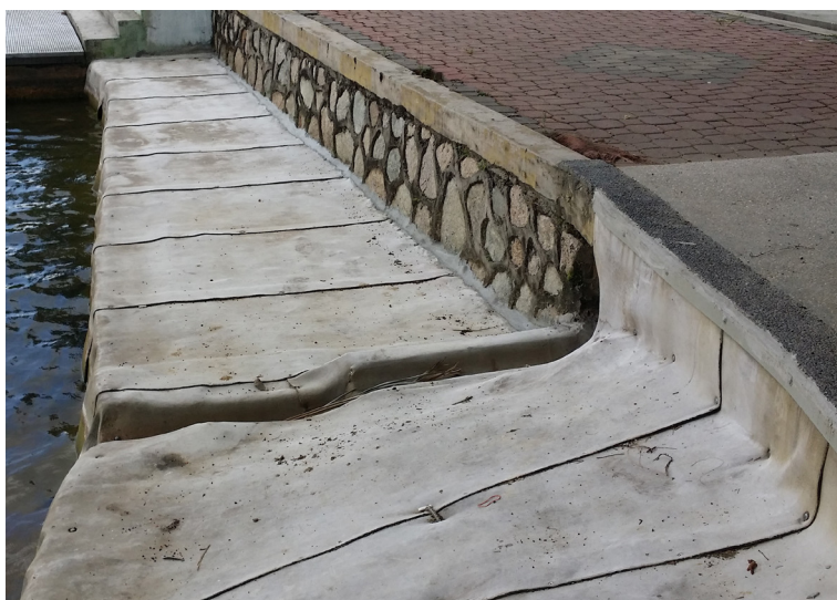
Poured concrete used to seal edges of CC and prevent further ingress
