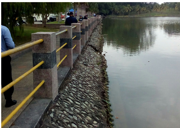
Original rip-rap slope sections
