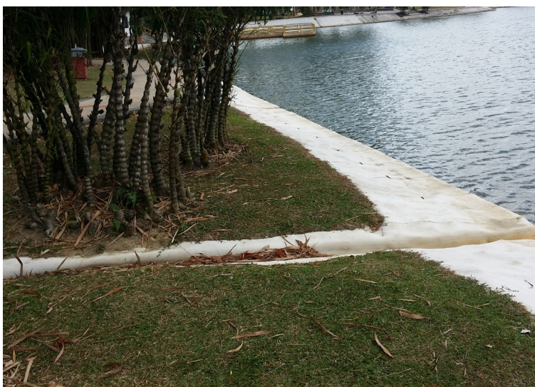
CC buried in anchor trenches to preserve grassy areas above slope
