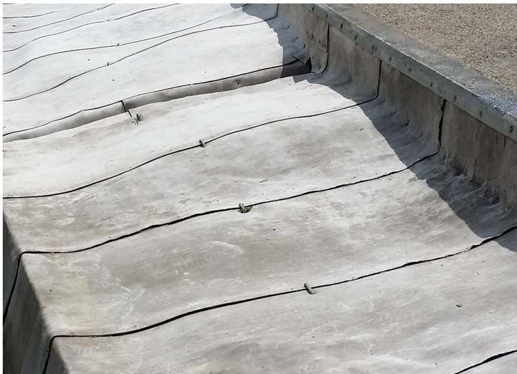
Ground pegs and concrete wall plugs were used to fix the CC
