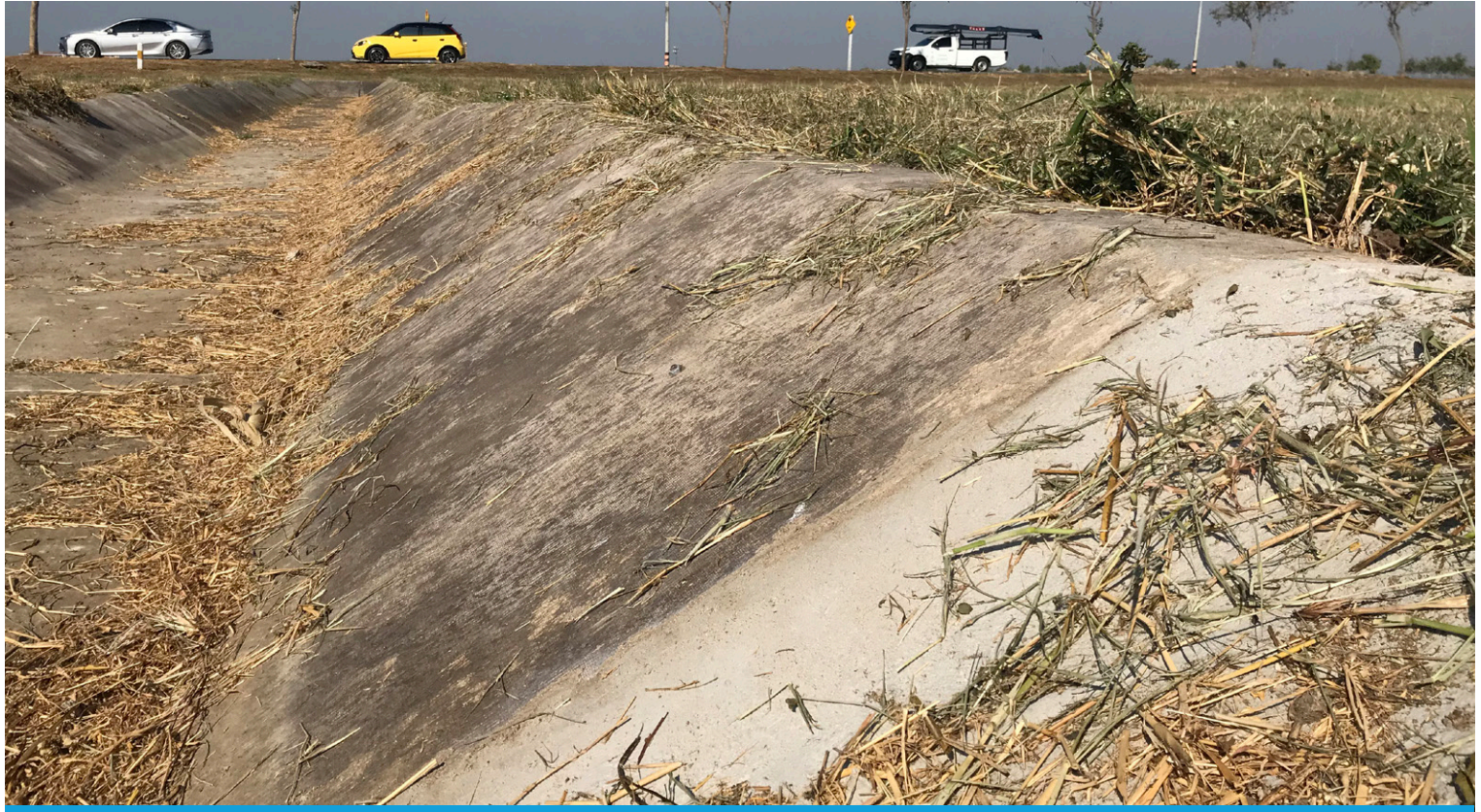
Completed installation and CC to concrete termination point
