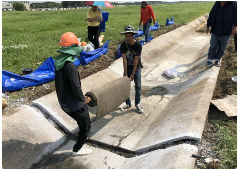
Preparing for deployment following removal of concrete section
