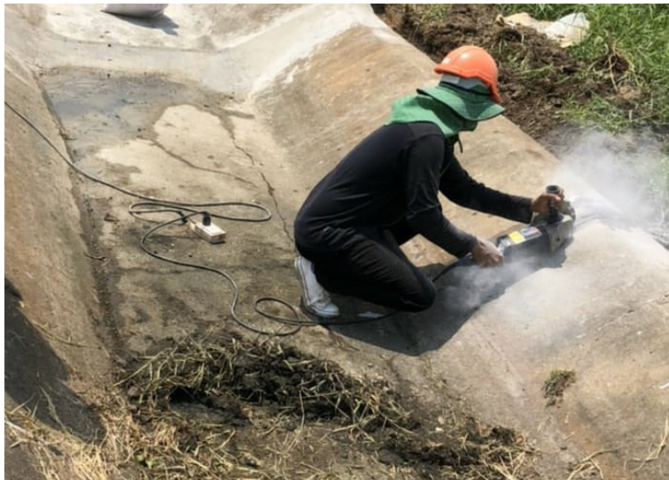
Angle grinder used to remove section of concrete for easier installation
