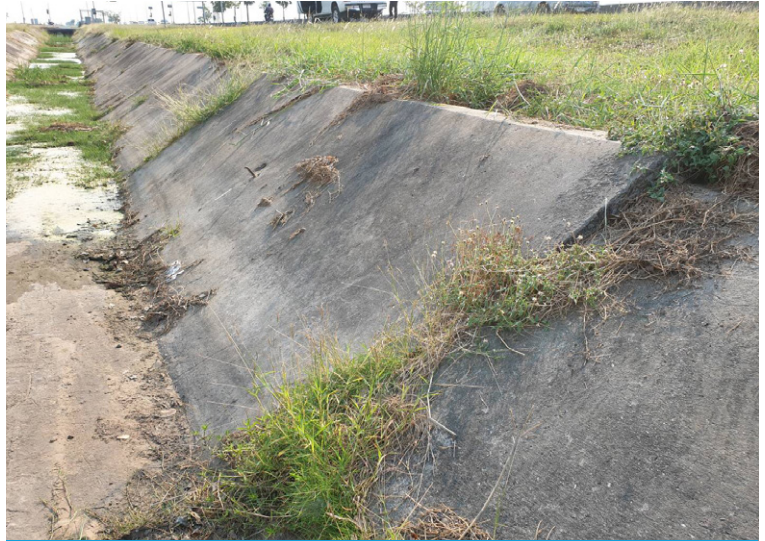
Channel had degraded and vegetation grew through cracks
