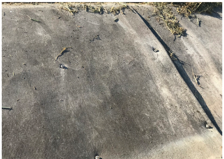
CC secured to concrete and at overlaps using SS screw anchors
