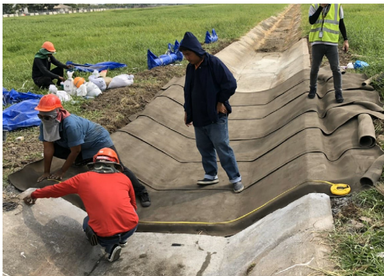
Deployment of CC batched rolls
