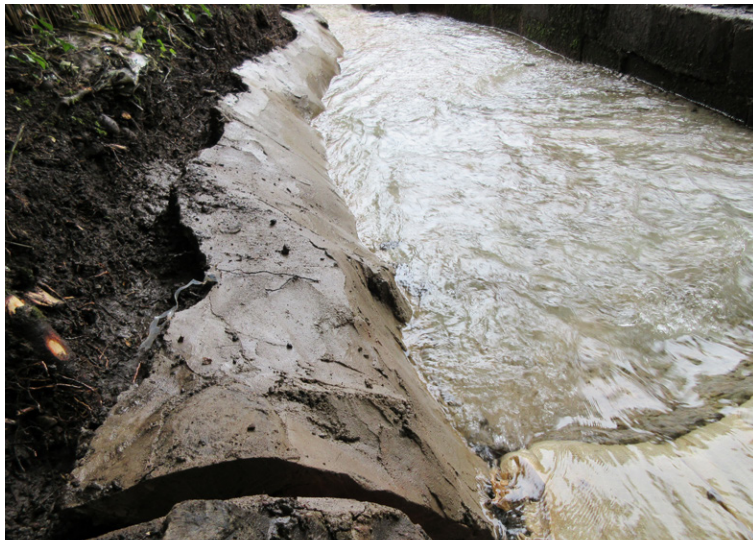
Channel side slopes coated with marine cement for a smooth surface
