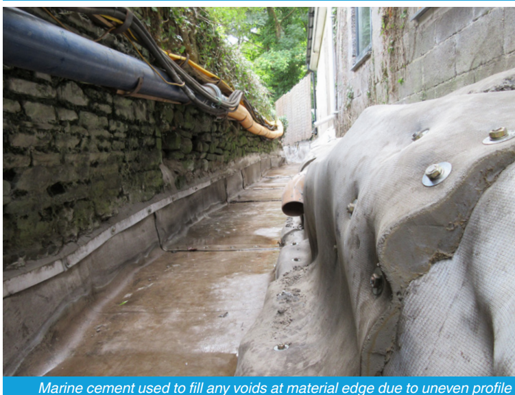
Termination of CC into anchor trench downstream
