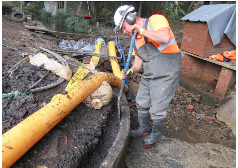
Anchor trenches were prepared by hand
