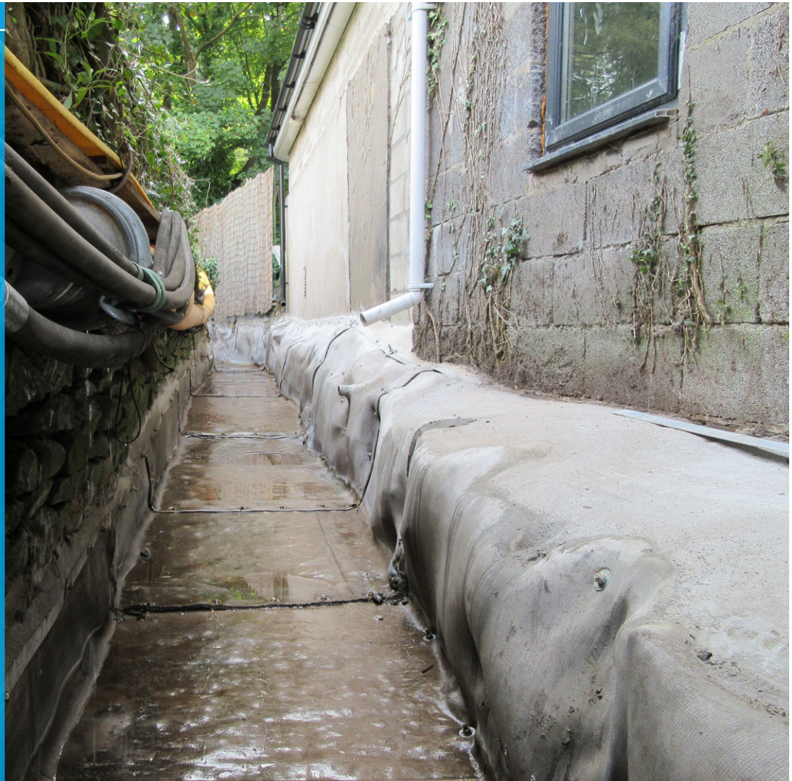
Completed CC remediation installation in Tongwynlais, Wales
