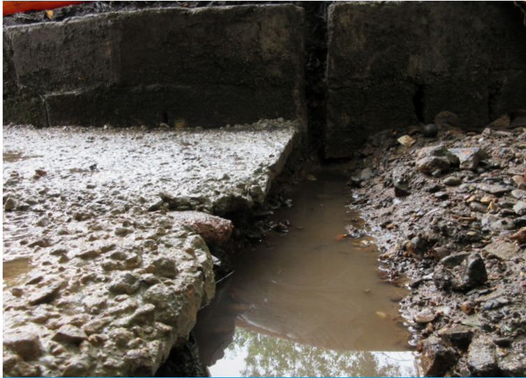
Anchor trench created for CC termination downstream
