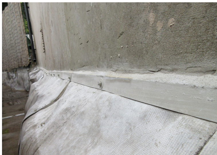
Termination of CC against outer wall of houses
