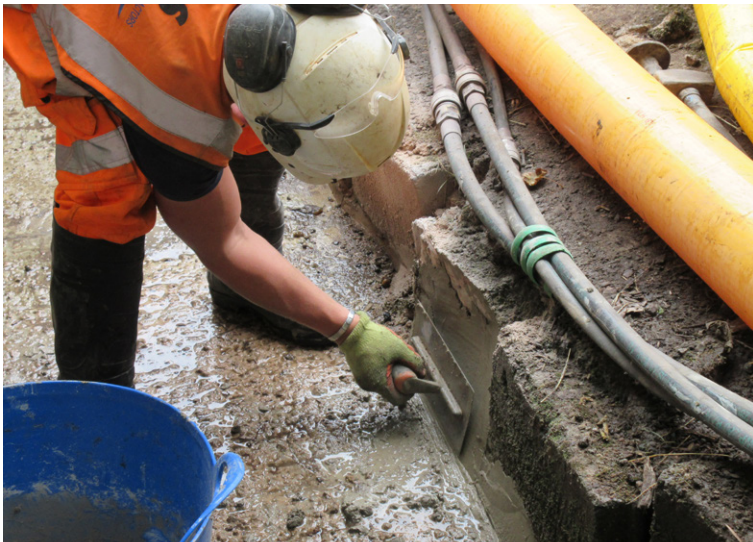
Marine cement used to fill voids in uneven blockwork
