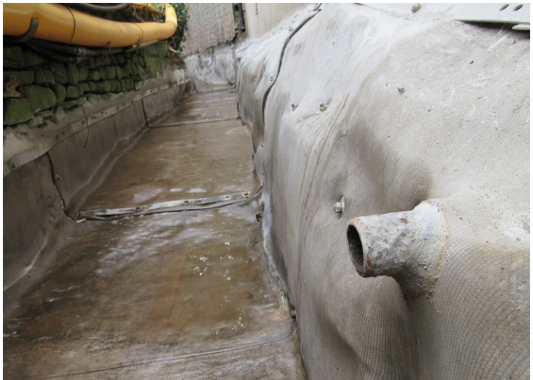
CC was cut to accommodate new and existing protruding pipework
