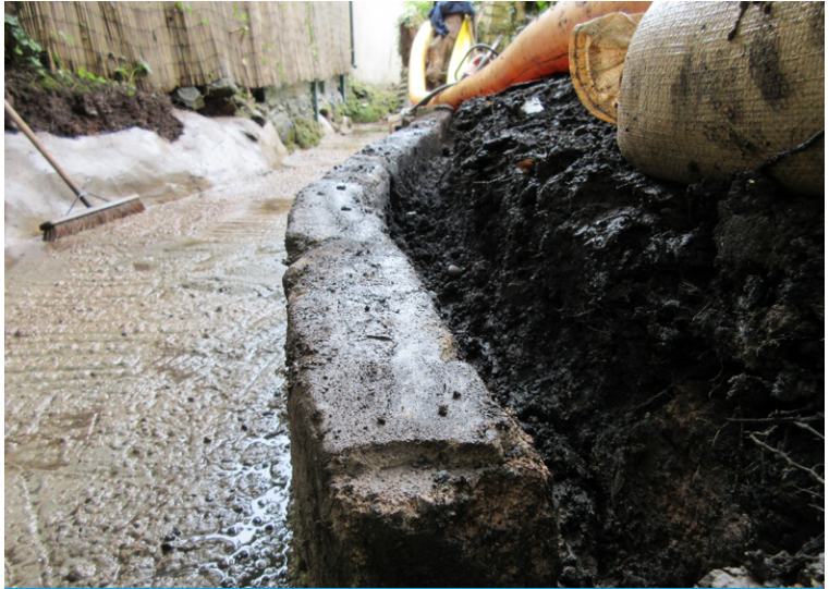
Anchor trench and brushed poured concrete finish for invert
