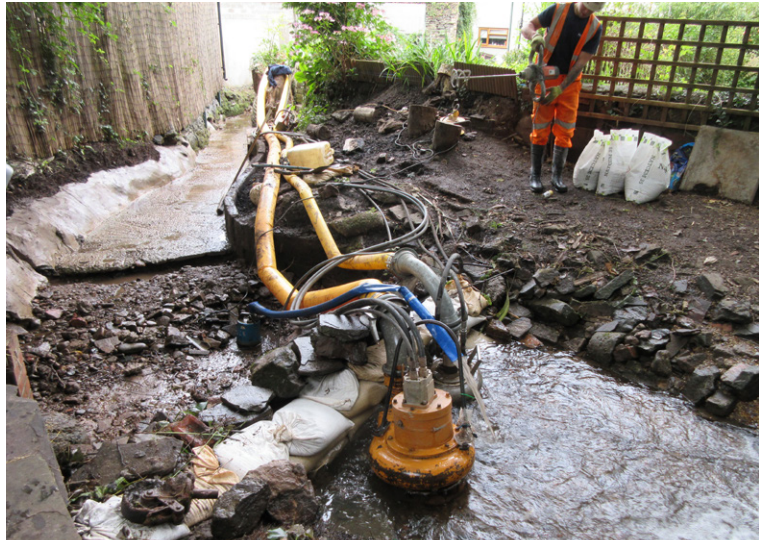
Water was overpumped to allow works to be carried out
