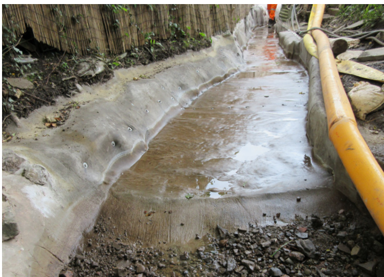
Termination of CC into anchor trench downstream
