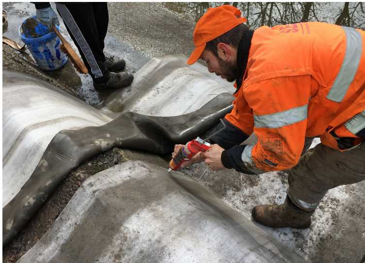
Clearfix was used to fix the CC material overlaps
