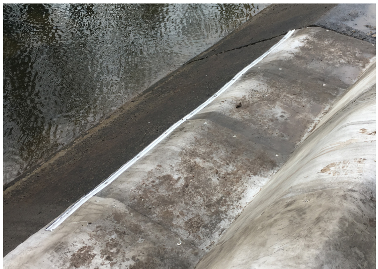
The bottom edge of the CC was fixed using bolts and a steel clamping strip
