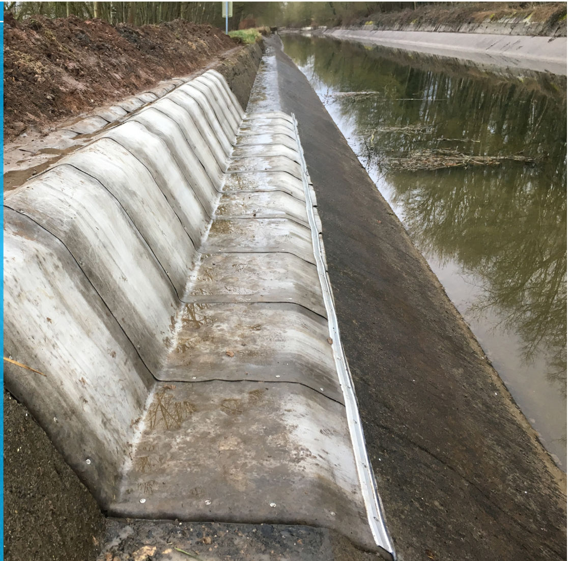
The completed canal remediation trial installation in Tonnoy, France
