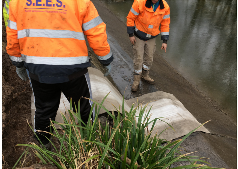
CC was laid transversely down the failing concrete bank
