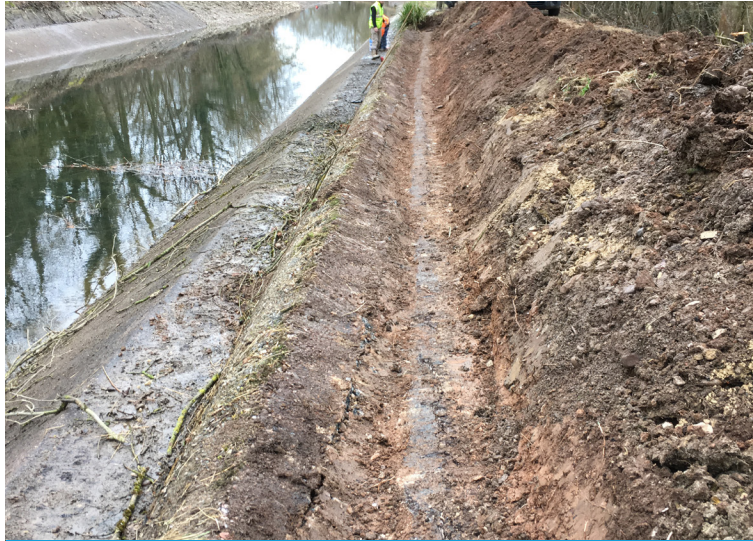
An anchor trench was dug above the failing concrete prior to installation
