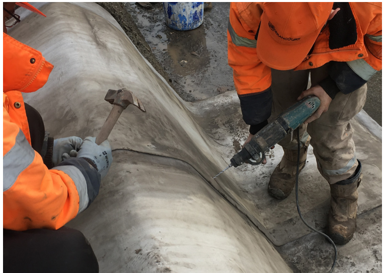
Holes were drilled through the CC and concrete before bolts were inserted
