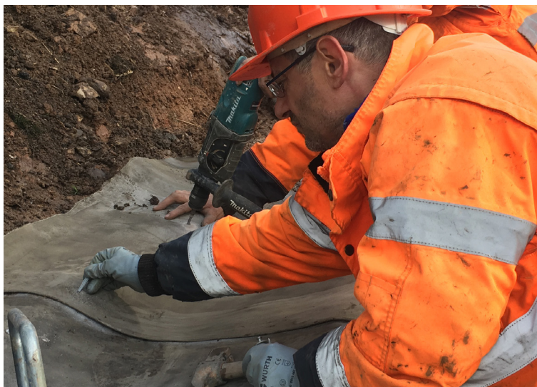
Insertion of the expansion bolt through the CC and into the drilled concrete
