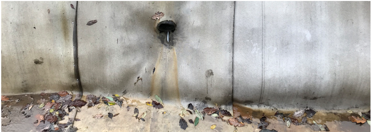
The flexibility of CC allowed the team to easily work around existing pipework
