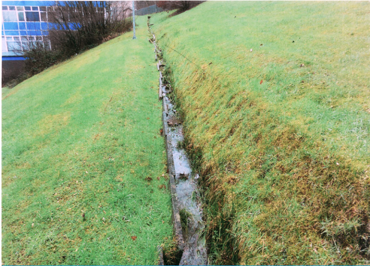
Loose concrete slabs were a H&S risk and decreased efficiency of the channel
