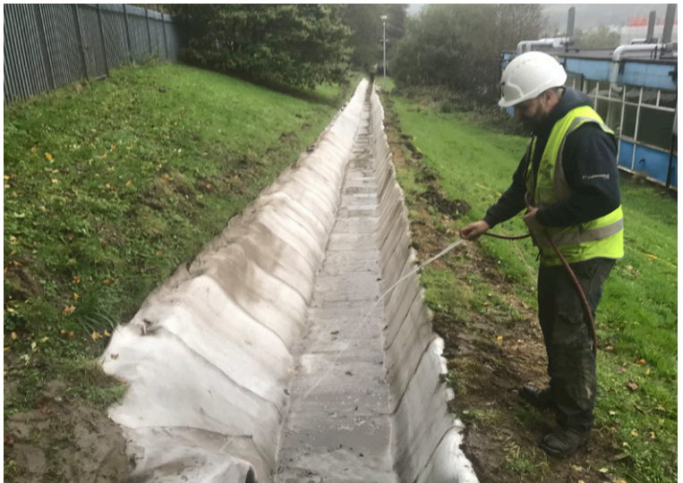
Once installation was completed, the CC was hydrated
