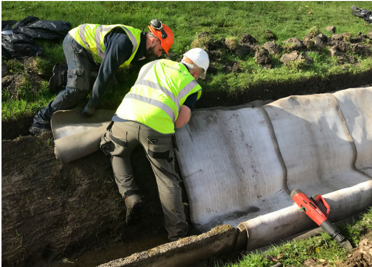
The leading edge of the CC was pegged in the embankment anchor trench
