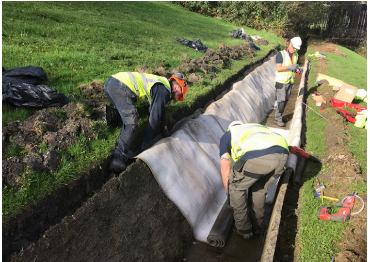
The CC was laid transversely with overlaps measuring 100mm
