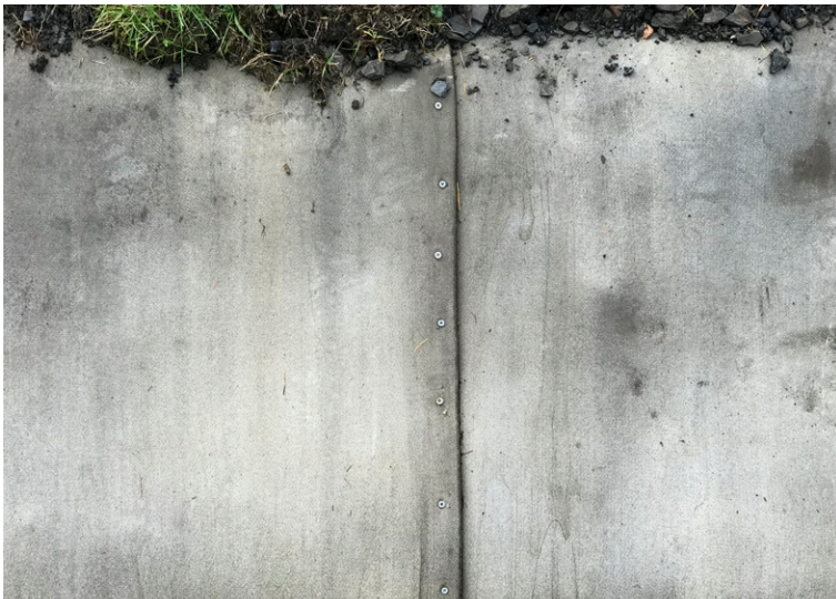
Joints were fixed using screws or Hilti shot-fired nails
