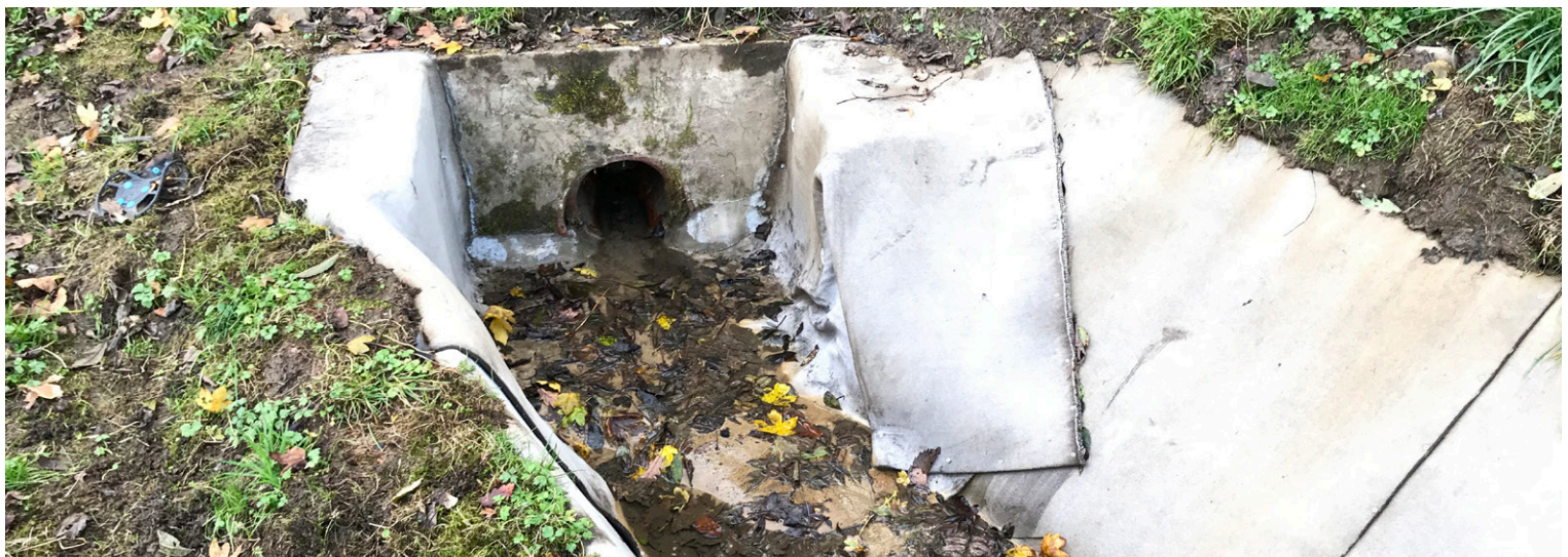
Termination of CC at a headwall
