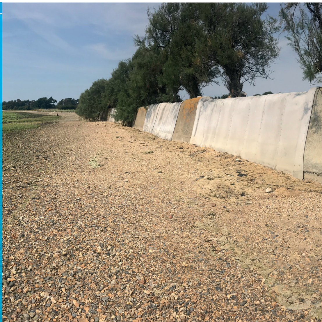
Completed sections of seawall repair installation
