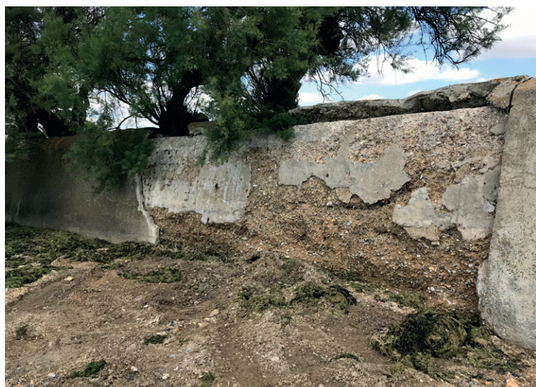
Section of damaged sea wall
