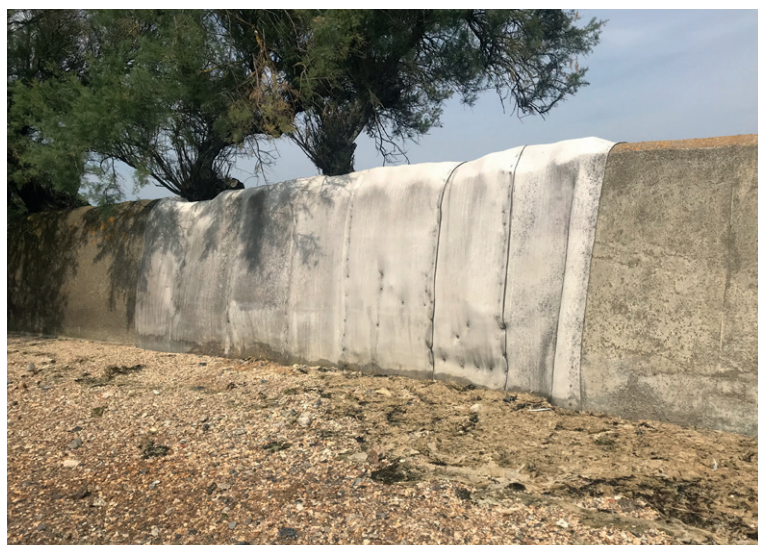
Vertical layers of CC used to cover damaged sections
