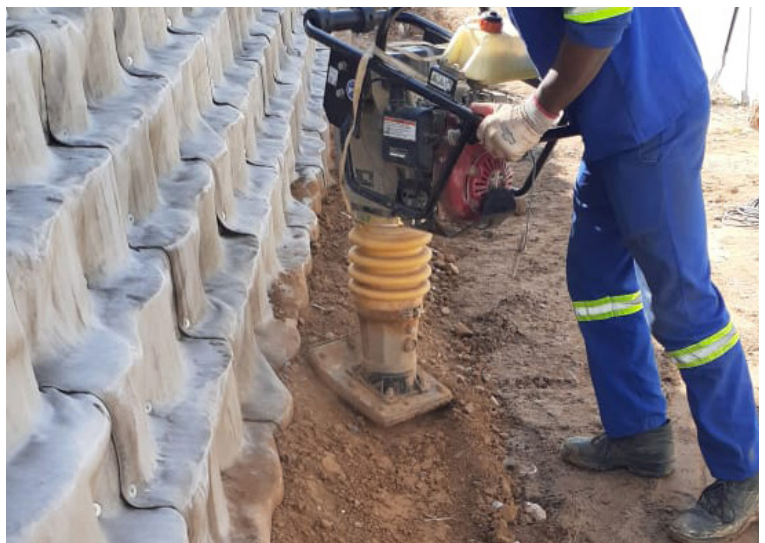
Compacting filled anchor trenches with mechanical rammer
