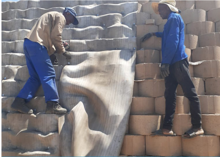
Lengths of CC installed vertically down wall face
