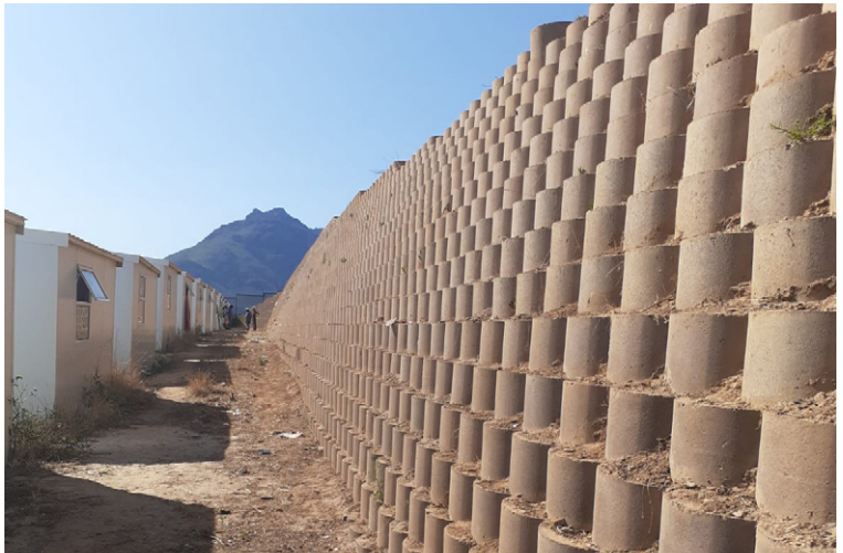
Dry stack wall prior to CC installation
