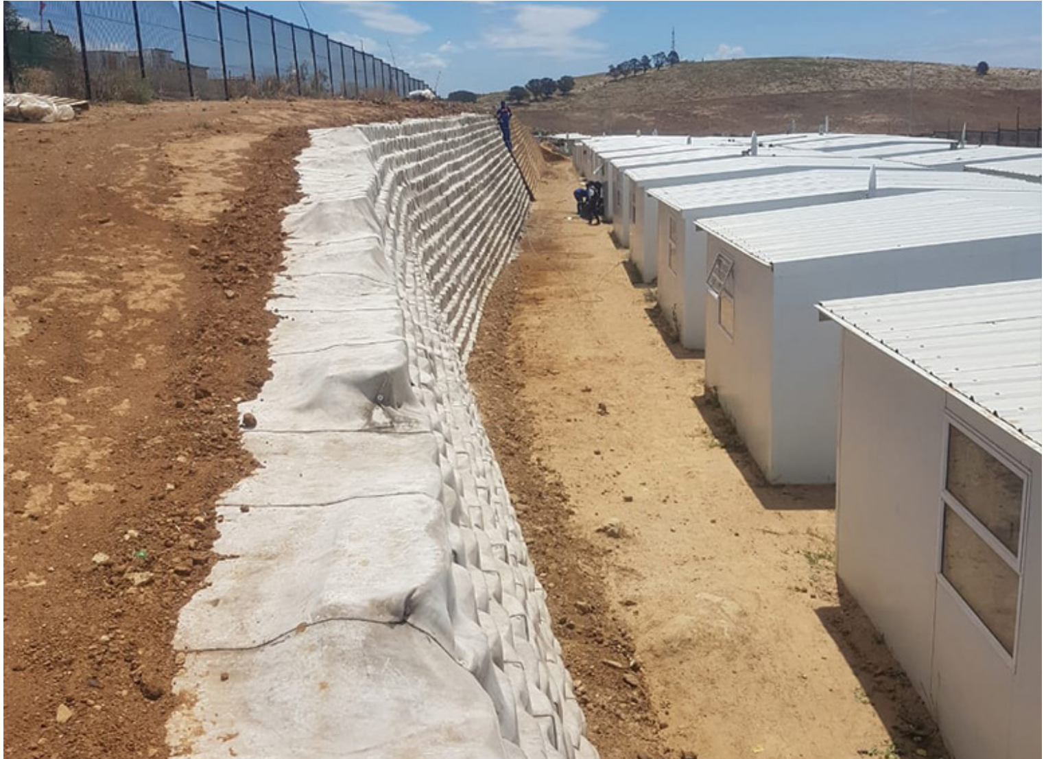
View of completed CC installation from top of dry stack wall
