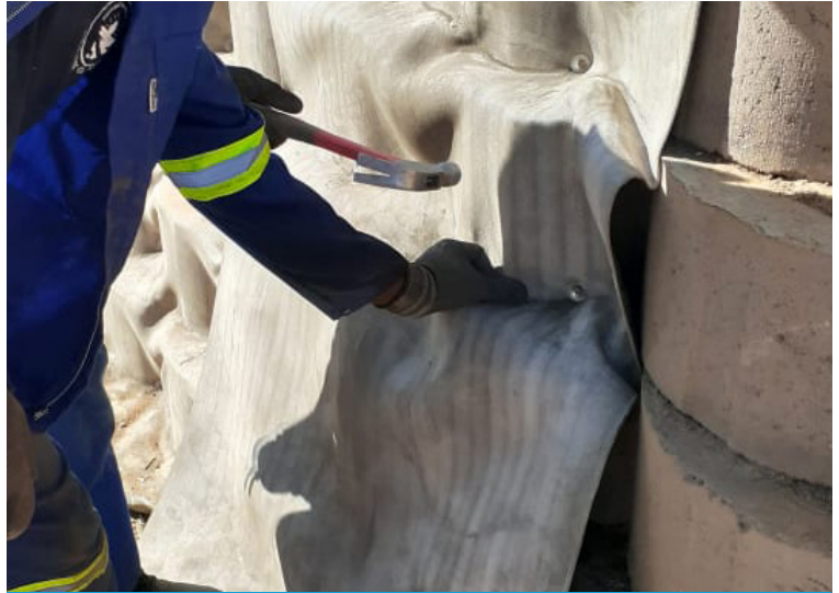
CC secured to dry stack wall using wedge anchors
