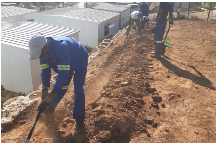
Preparation of anchor trenches
