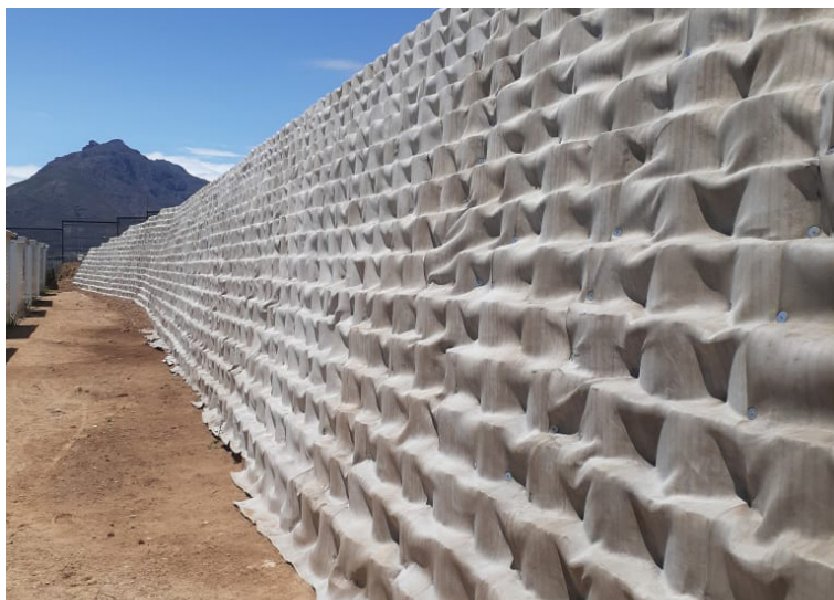
Completed CC installation prior to backfilling of anchor trenches
