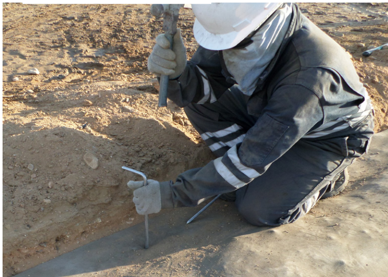
Pegs were used to fix the CC in the trenches
