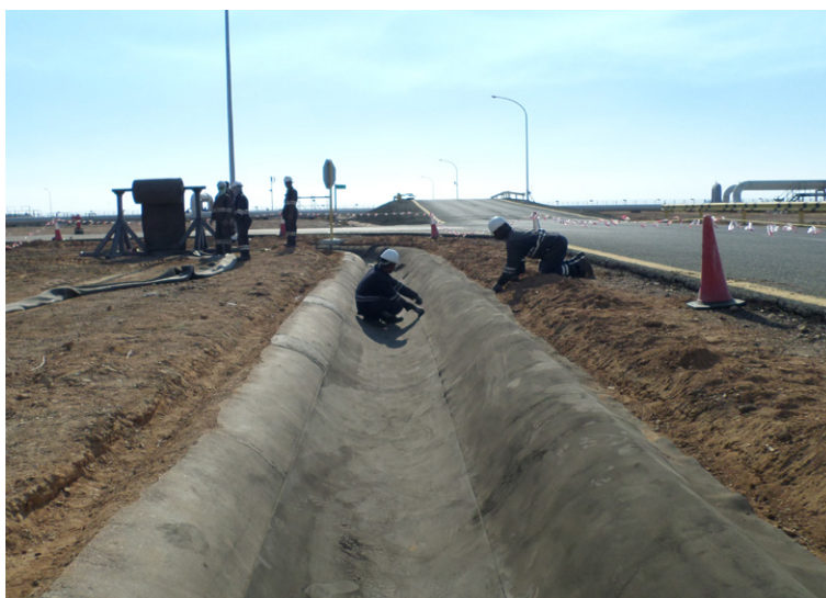
CC8™ was laid longitudinally down either side
