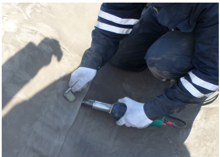
CC was sealed with a hot air gun before fixings were applied
