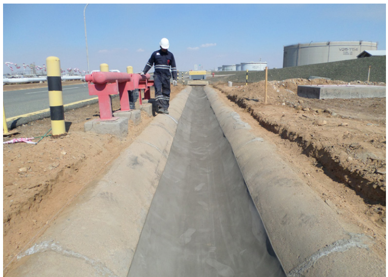
CC5™ was laid down the middle of the channel
