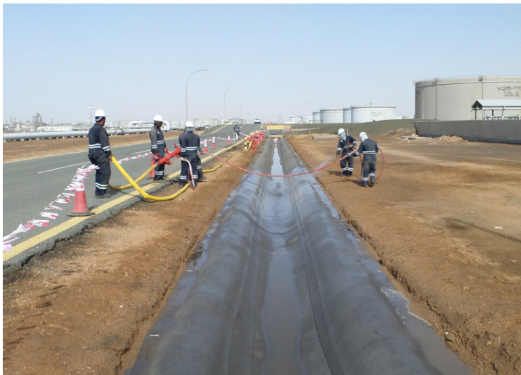
CC was hydrated using a fire hose
