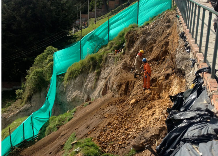
Slope instability and slip posed a risk to an adjacent construction project
