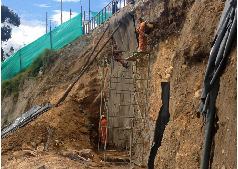
CC8, unlike shotcrete, was able to be installed without heavy plant
