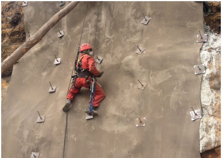
Soil nails with 200mm plates were used to secure CC to the slope
