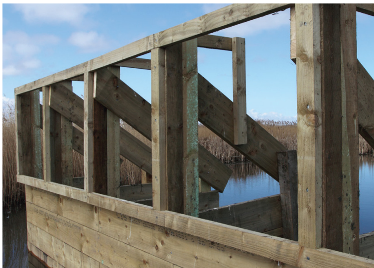
Timber frame prior to installation of CC8
