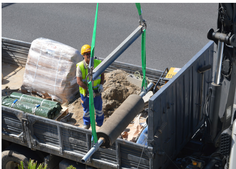
Batched rolls delivered to site and mounted onto a spreader beam
