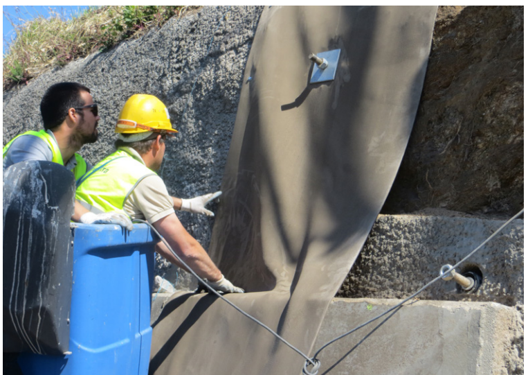
Anchor plates used to profile CC
