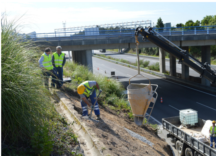
Large voids filled with aggregate
