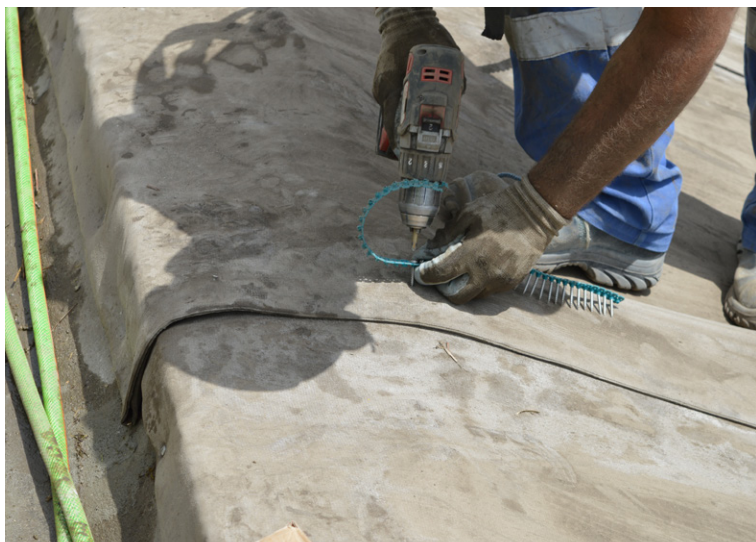
Overlaps were screwed at 200mm centres
