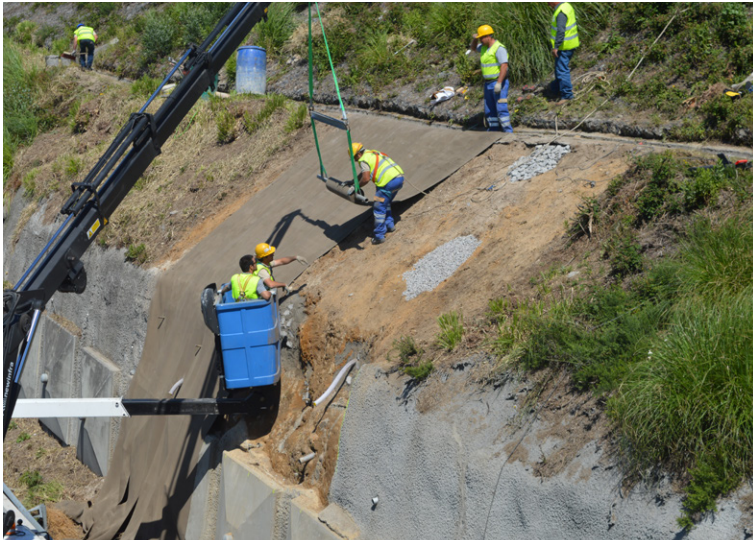
Subsequent layers overlap previous by 100mm
