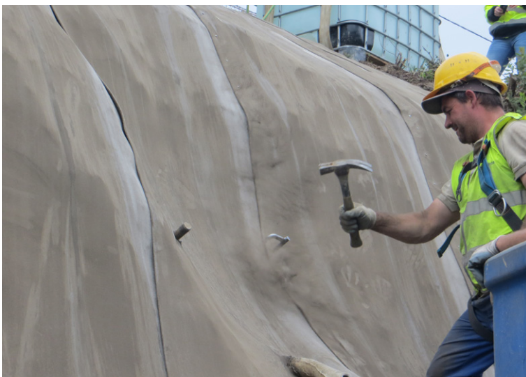
Ground pegs inserted through the overlap
