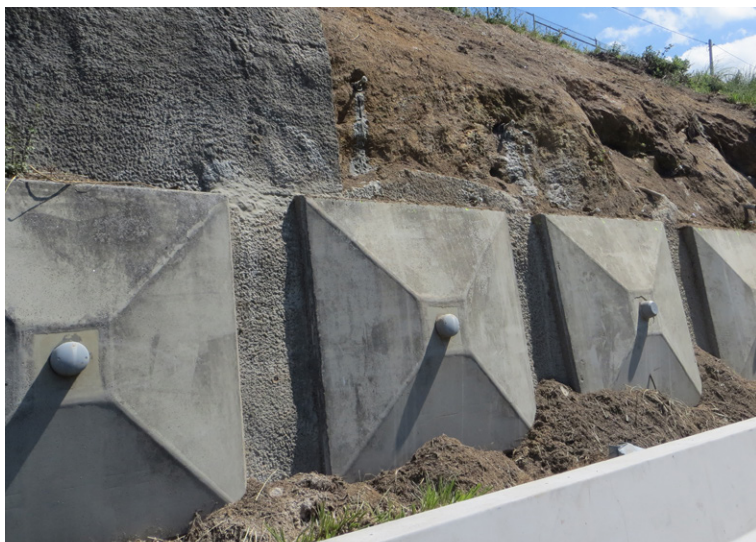
Erosion occurred under the previous shotcrete installation
