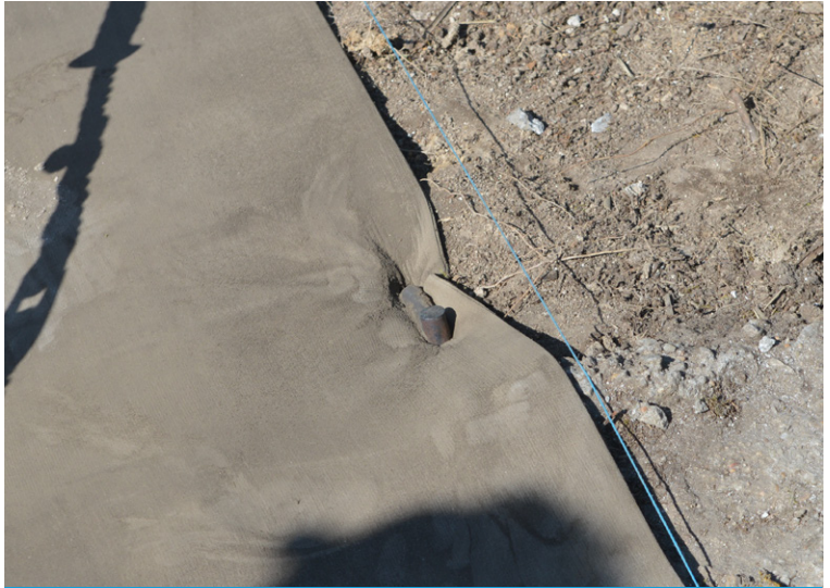
Fixed to substrate with ground pegs
