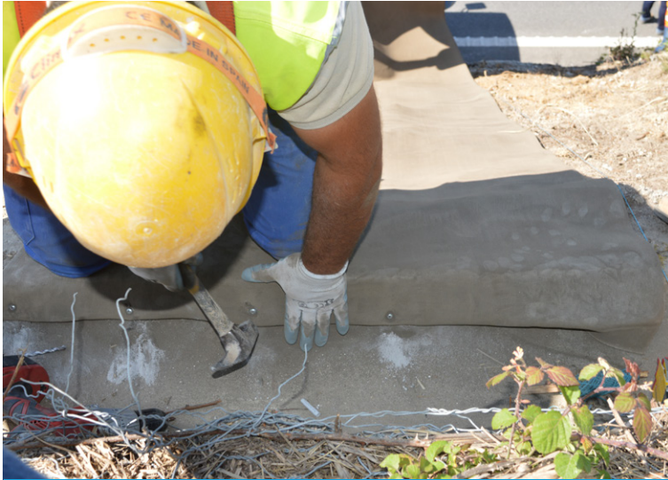
Fixing to existing concrete channel with wedge anchors
