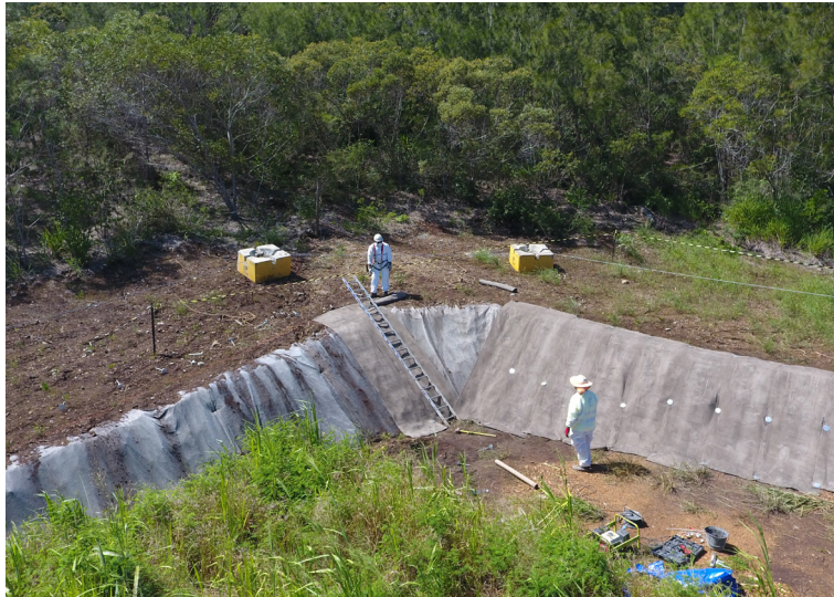
CC laid longitudinally from crest to toe of slope
