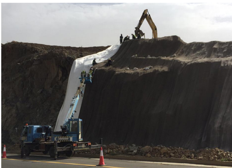
CC's flexibility allowed for close contact between the slope and material
