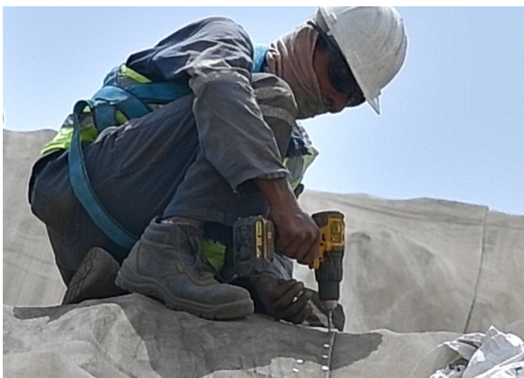
Joining overlaps using stainless steel screws
