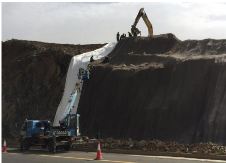
CC's flexibility allowed for close contact between the slope and material
