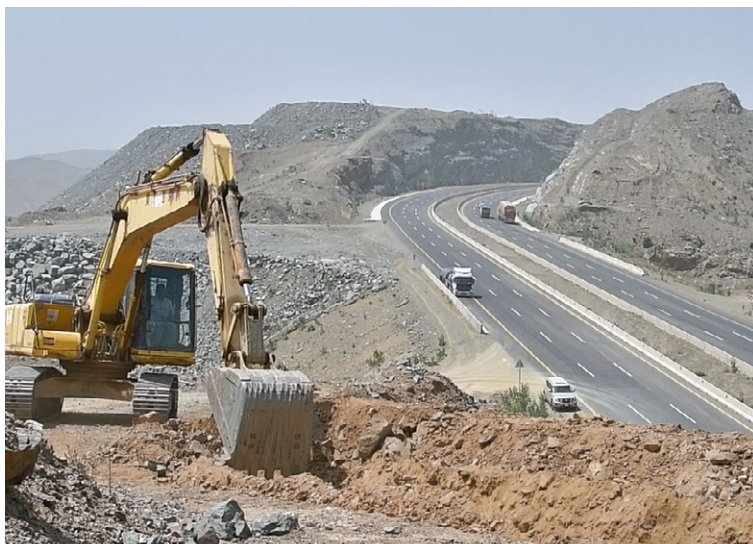
Anchor trenches were dug mechanically at the crest and toe
