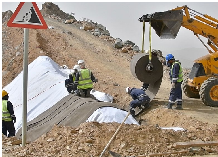
Deployment of CC bulk rolls from the slope's crest
