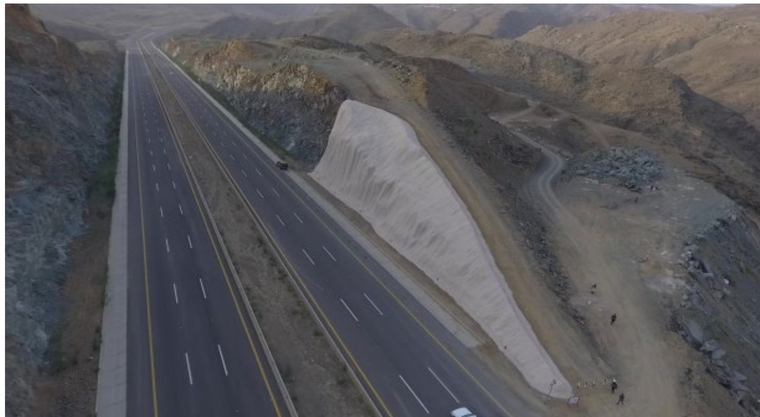
CC was painted following install to allow the material to blend in more successfully with the surrounding environment
