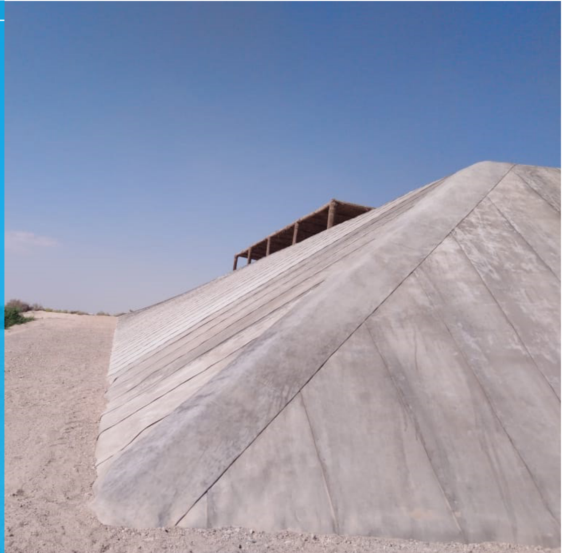
Completed installation following hydration and backfilling of anchor trenches
