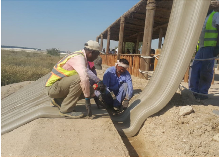
CC deployed and captured in anchor trench
