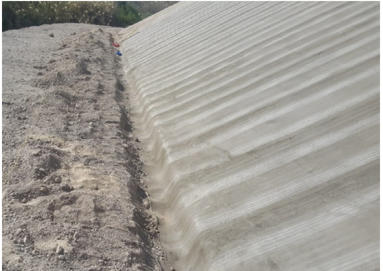
Material pegged into anchor trench at toe
