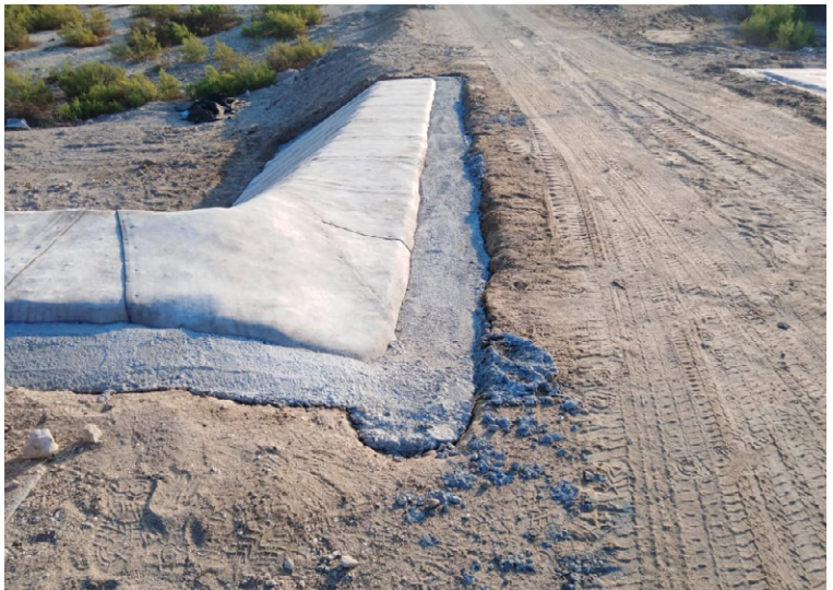
Anchor trench at crest backfilled using poured concrete
