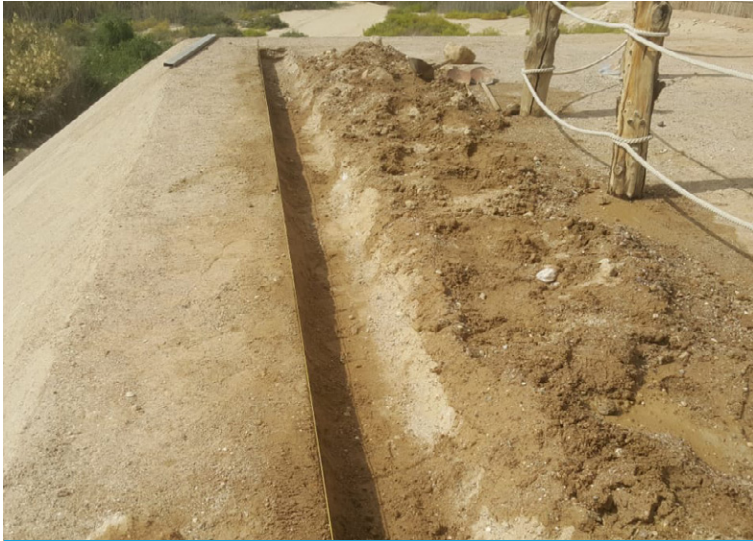
Anchor trench prepared
