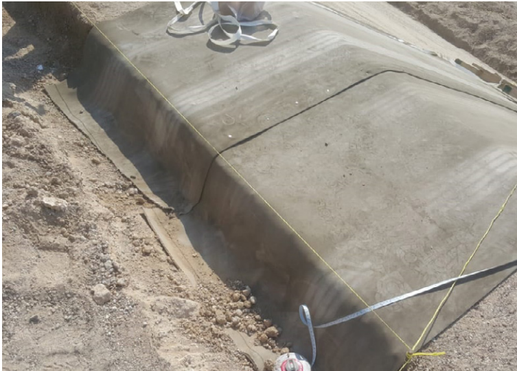
Material pegged into anchor trench at crest
