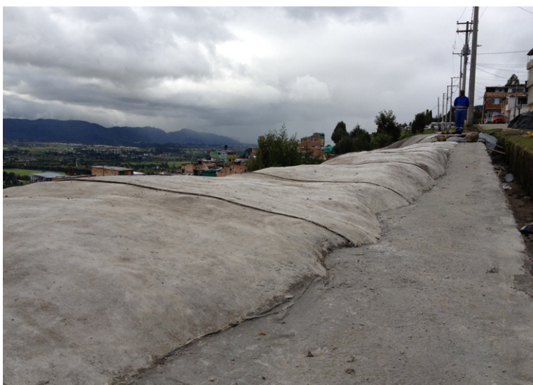
Crest anchor trench backfilled with poured concrete
