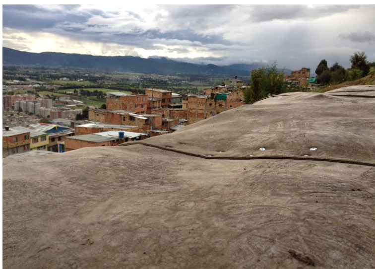
CC overlaps jointed using screws
