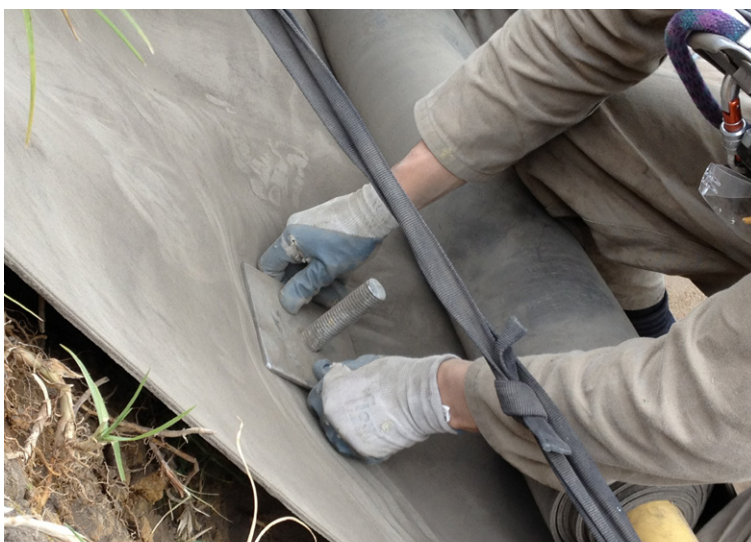
CC fixed to slope face using steel plats and soil anchors
