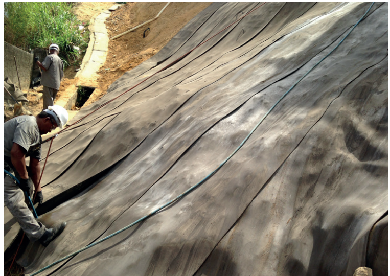
Hydrating under the overlap
