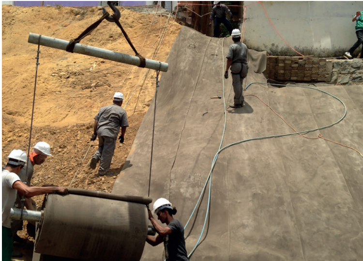
CC spooled down the slope
