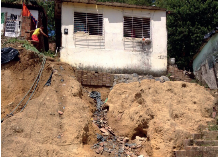
Extensive erosion of the slope
