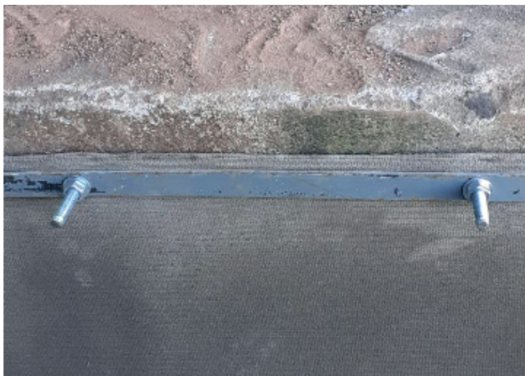
CC terminated around concrete plinths using clamping bar
