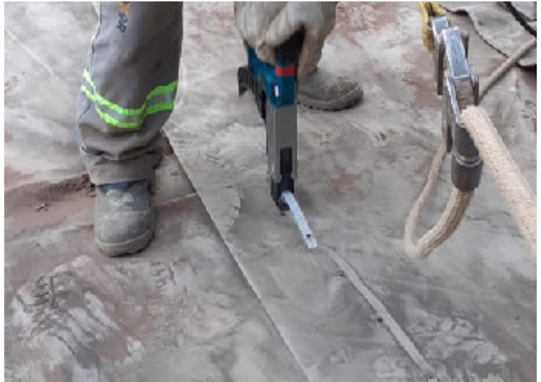
Overlapped edges were screwed together using an auto-fed screwdriver
