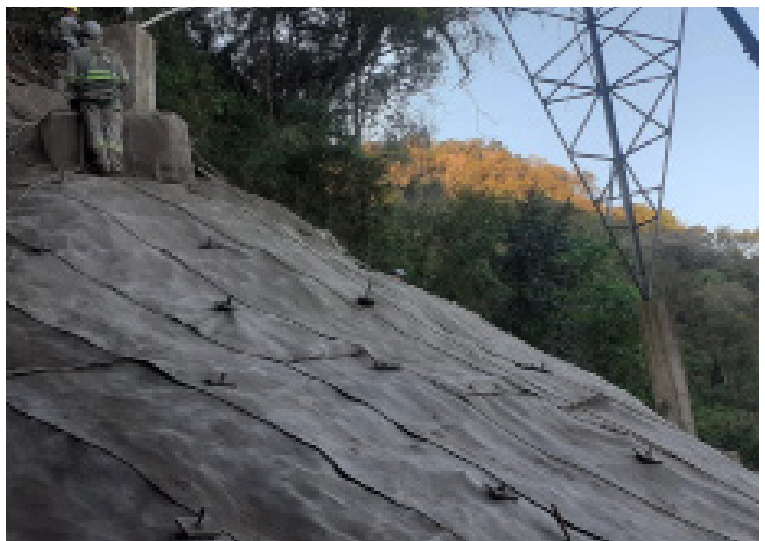
anchors and plates used to ensure CC conforms to the slope profile
