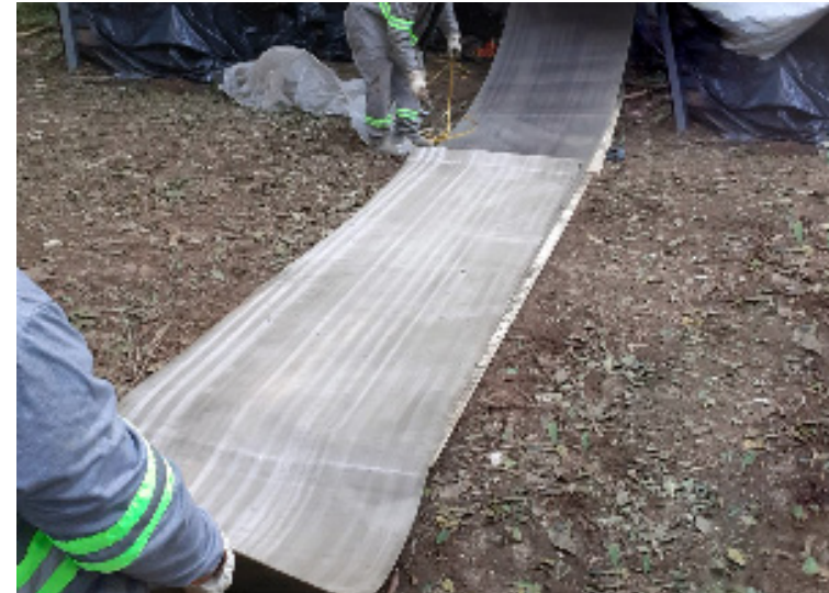
Bulk Rolls batched on site to suit handling limitations
