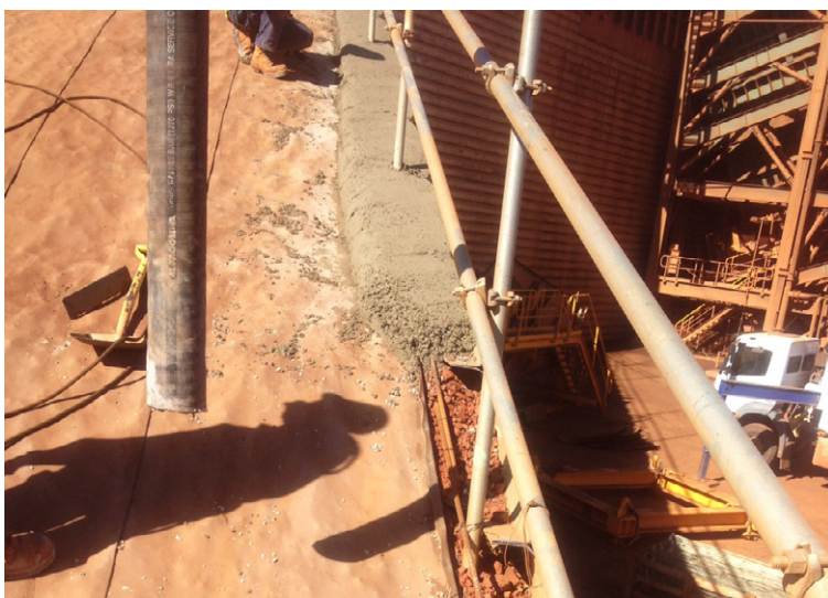
Concrete was poured along the edge adjacent to the wall
