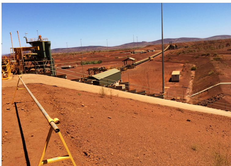
The CC5 was laid vertically down the length of the slope
