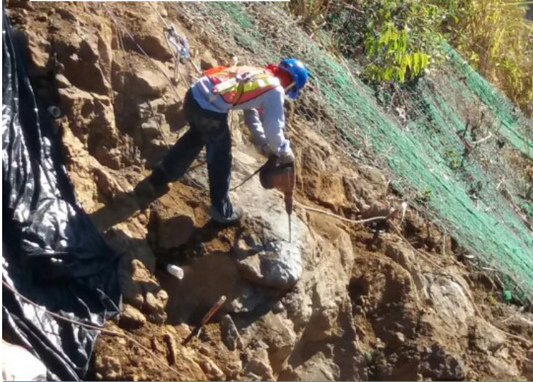
Inserting anchor bolts into the slope before installation
