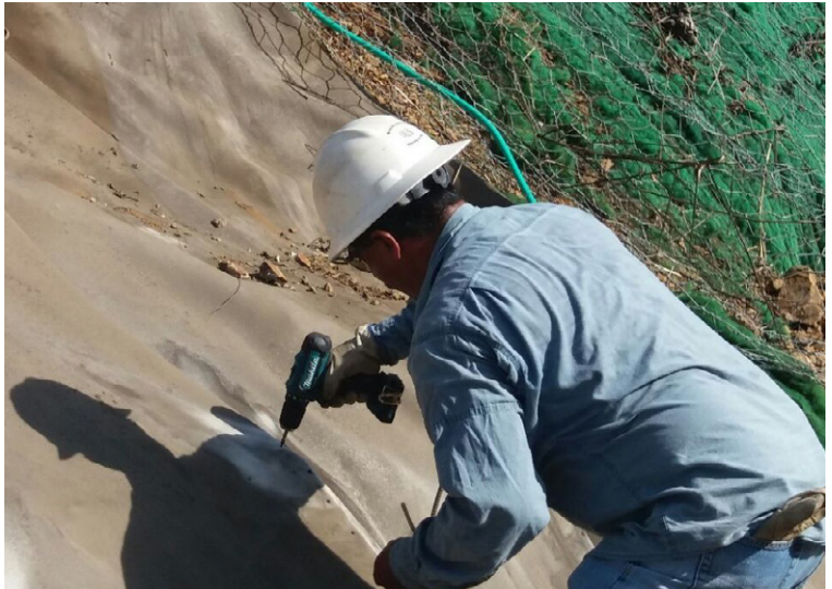
Screws were inserted at the overlaps to fix the CC
