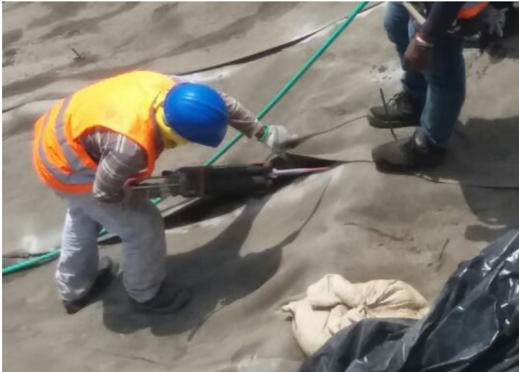
Epoxy sealant was used to seal overlaps of the CC and prevent ingress
