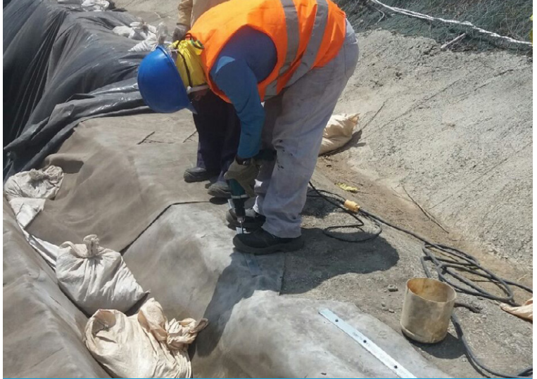
Steel bars and screws were used to fix the CC at the crest
