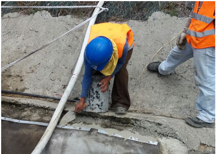
Cement was used to cover and seal the edges of the CC at the crest
