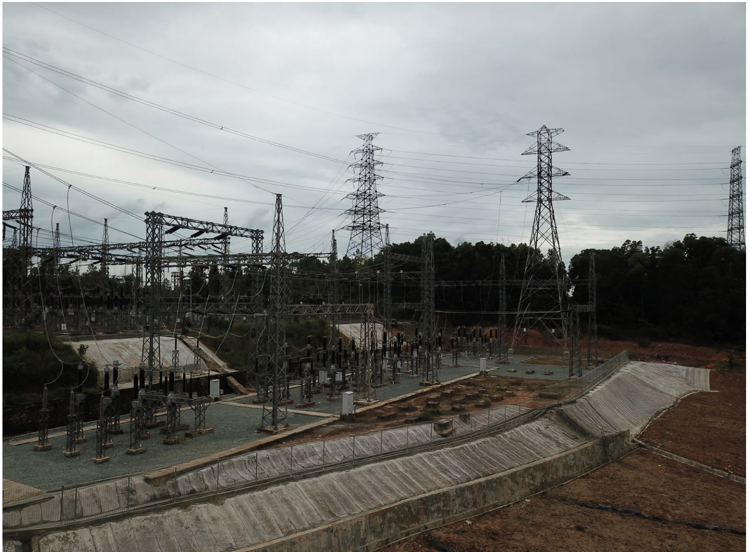
Completed channel and slope protection works
