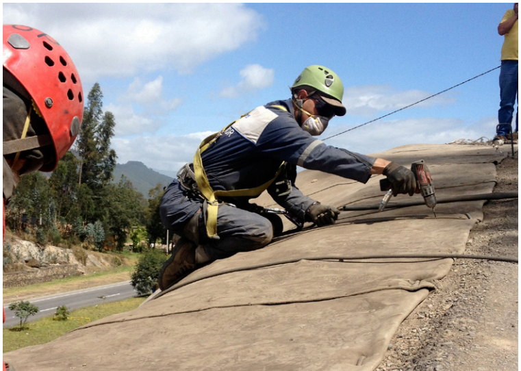
Adjacent layers of CC were overlapped by 100mm and screwed together
