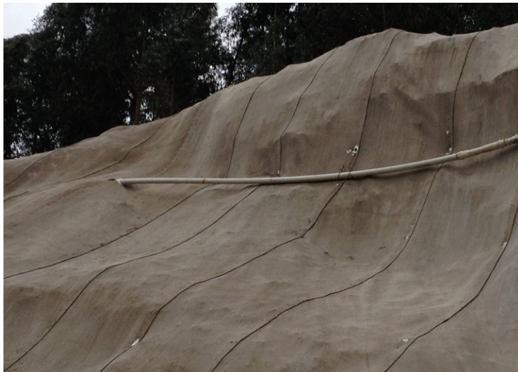
CC's flexibility follows slope profile to prevent voids forming below material
