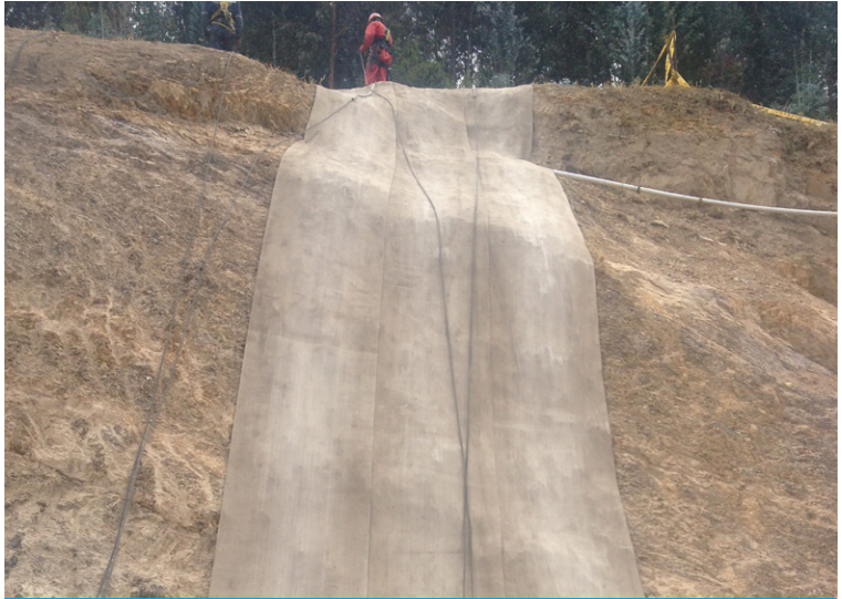
Spreader beam and climbing equipment were used to install CC
