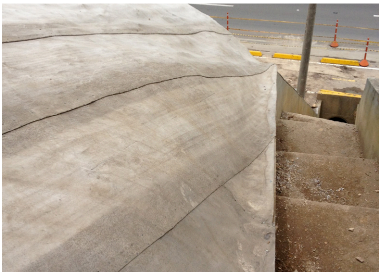
Completed section showing CC tailored around existing infrastructure
