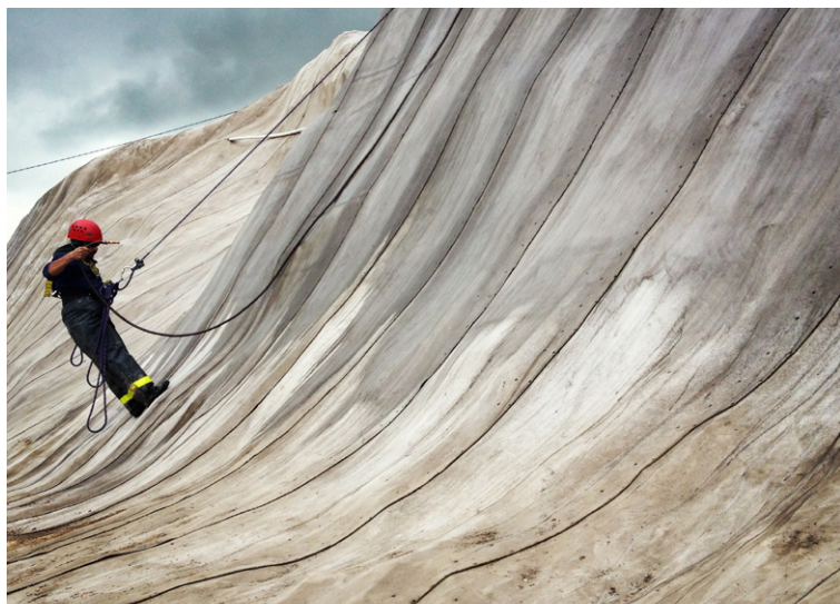
CC hydrated using hose and climbing equipment
