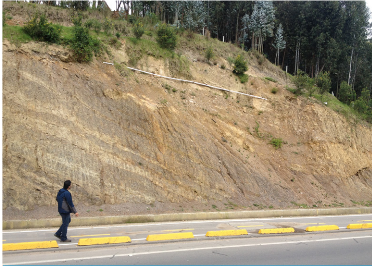
The slope prior to installation of CC, displaying signs of slip and erosion
