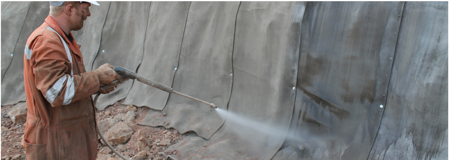
CC hydrated water from a dust suppression tank
