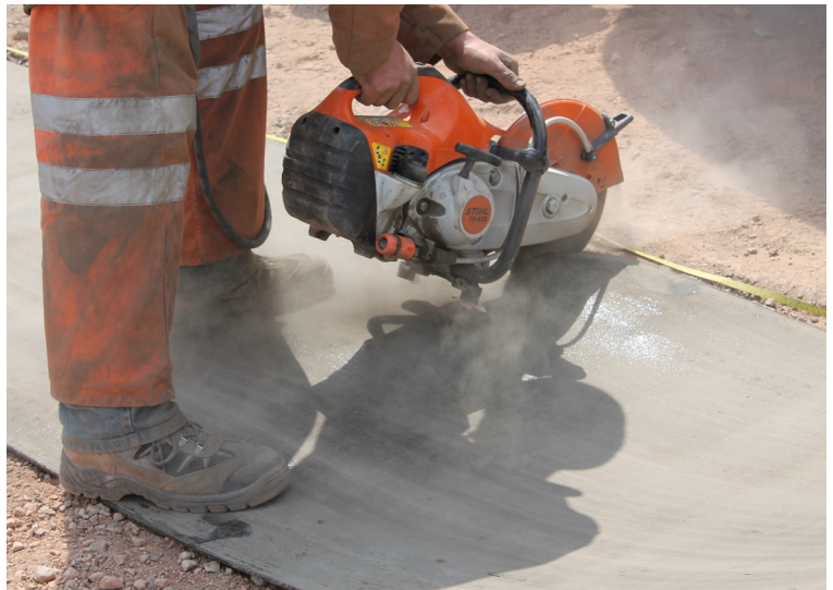
Unset CC8 was cut to length using a disk cutter
