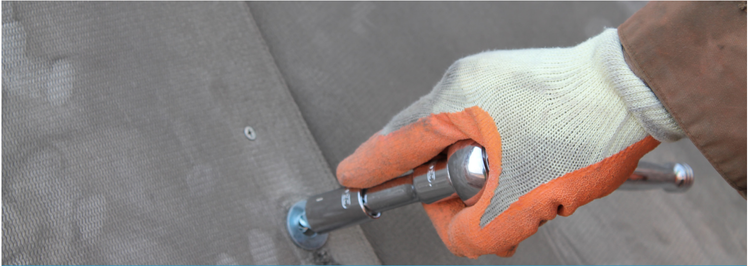
Rock bolts used to reinforce fixings
