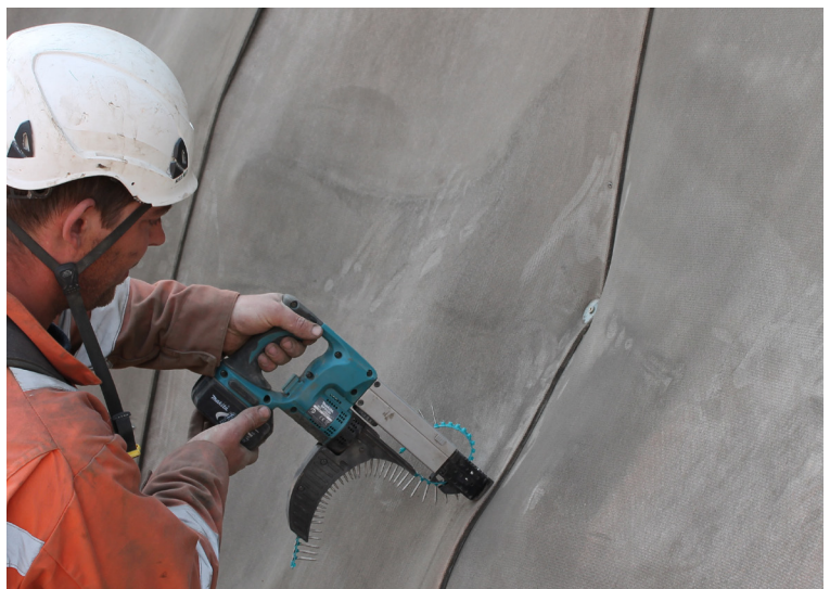
Overlapped CC edges fixed using auto-fed screw driver
