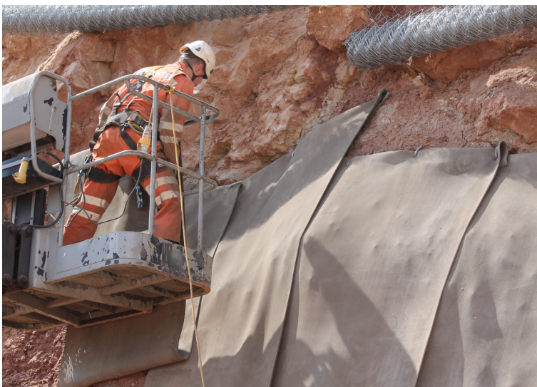
CC hung from top of rock surface using steel ground pegs
