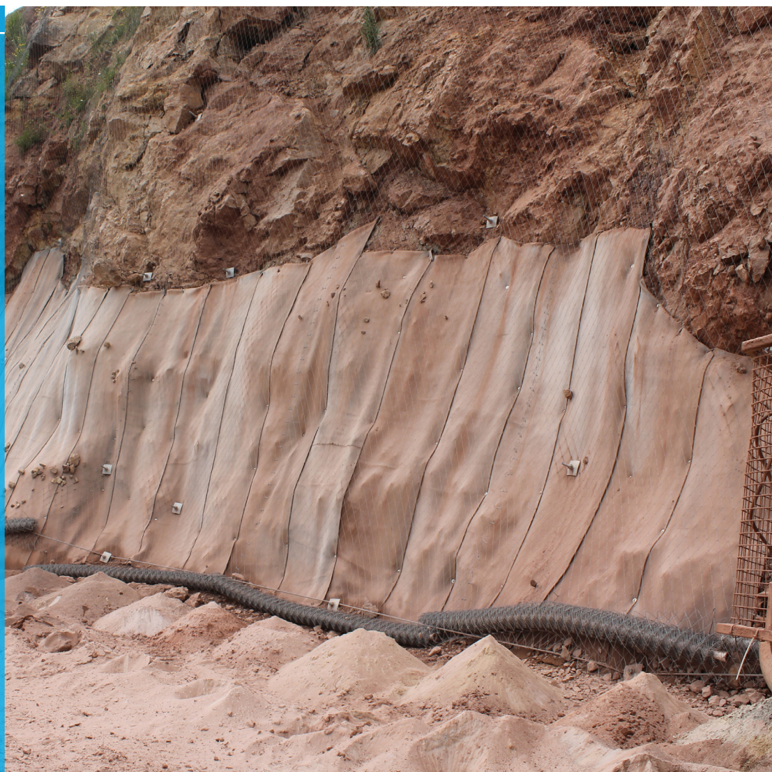
Completed section of slope lined with CC5
