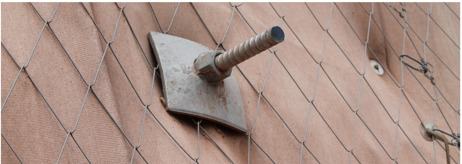
GEWI thread bar system with load bearing plates and nuts
