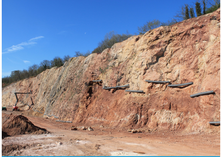
Quarry rock surface with unstable sandstone overburden prior to installation
