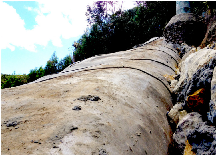
Anchor trench at top of slope backfilled with soil and rock for better stability
