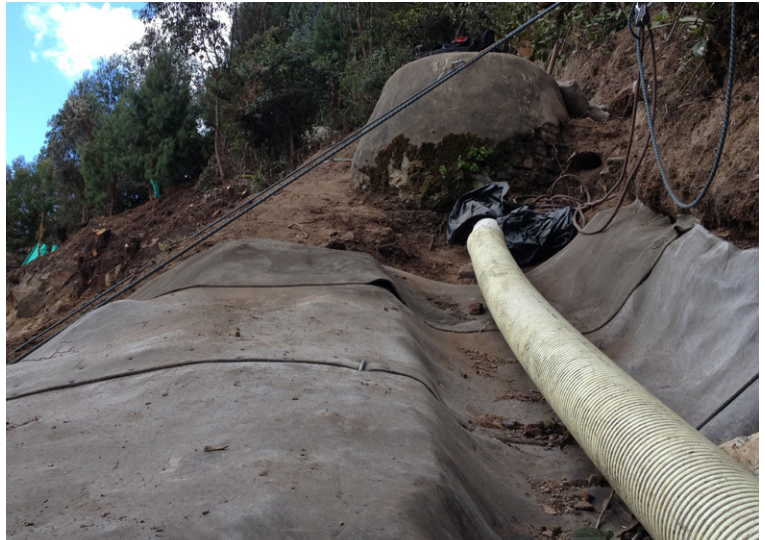
CC secured in anchor trench with ground pegs
