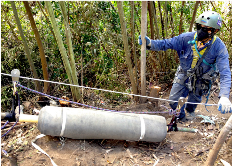
Pre-cut batched rolls of CC on rope mounted spreader beam
