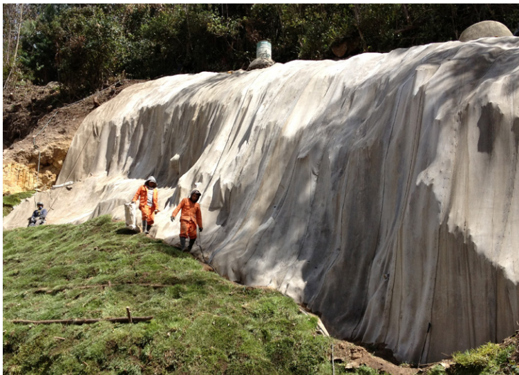
CC was able to conform to complex surface of slope
