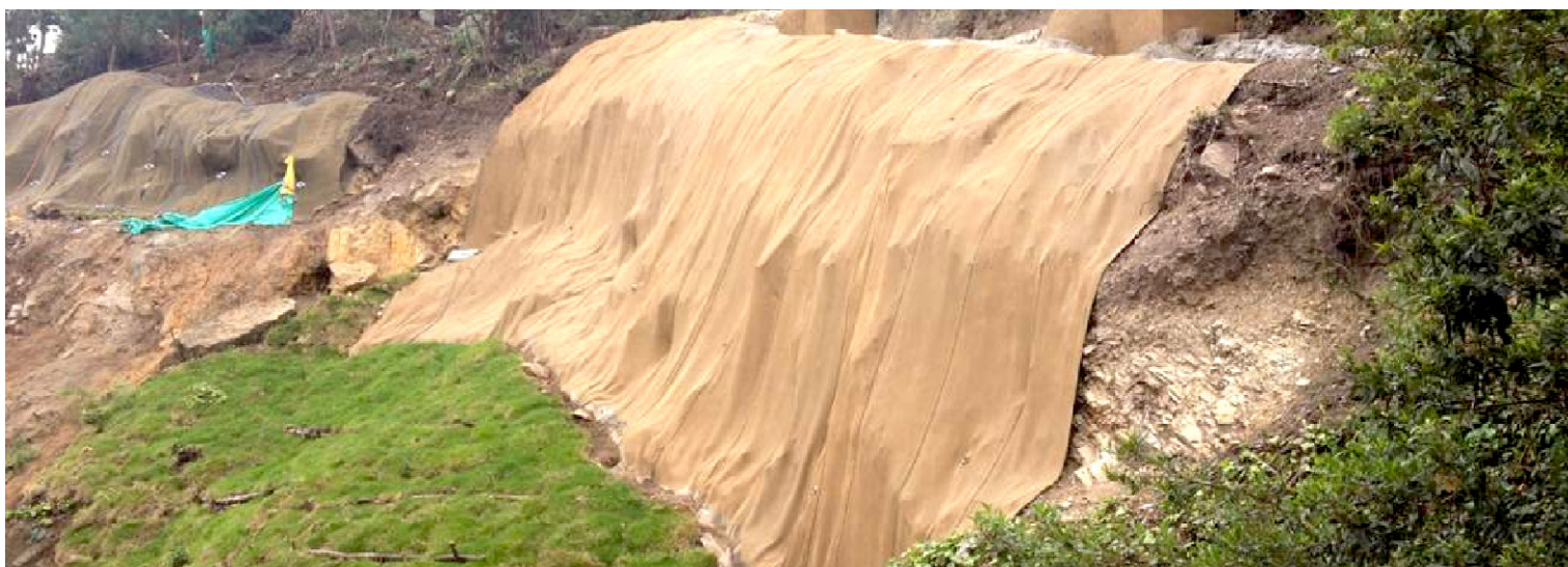
CC painted with standard masonry paint after installation
