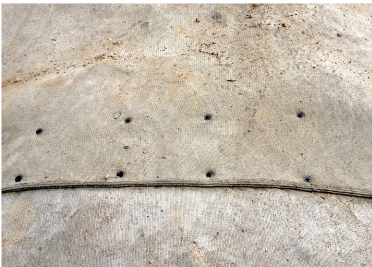
CC overlaps double screwed at 120mm intervals
