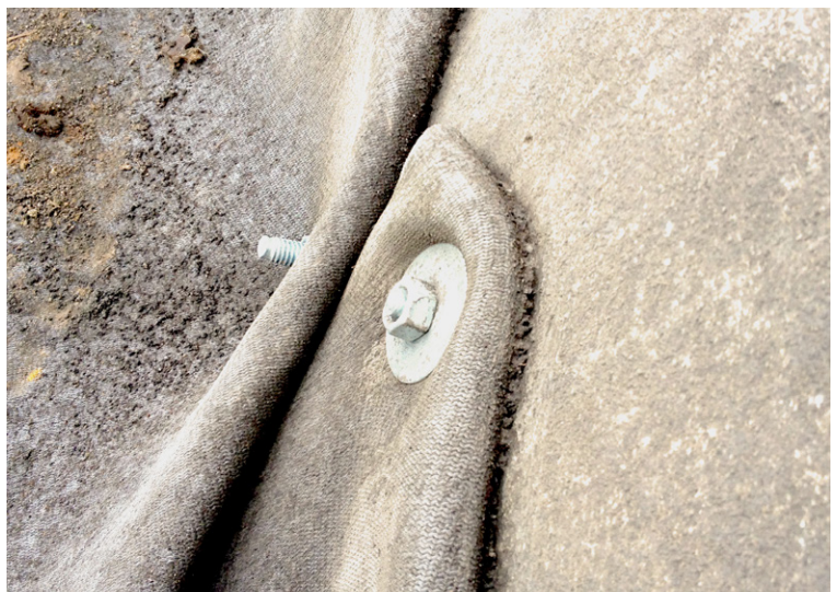
Expansion anchors used to close voids between CC and uneven profile
