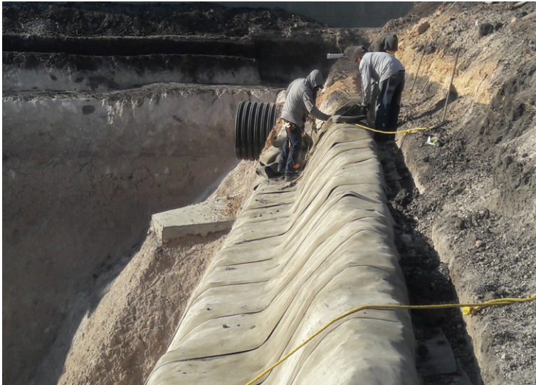
CC was anchored in a trench and covered with concrete for reinforcement
