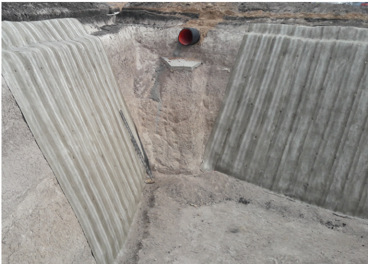
CC5™ was laid vertically down the slope
