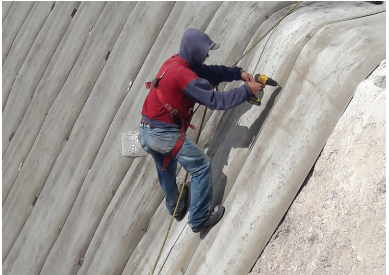
CC was secured at regular intervals with screws
