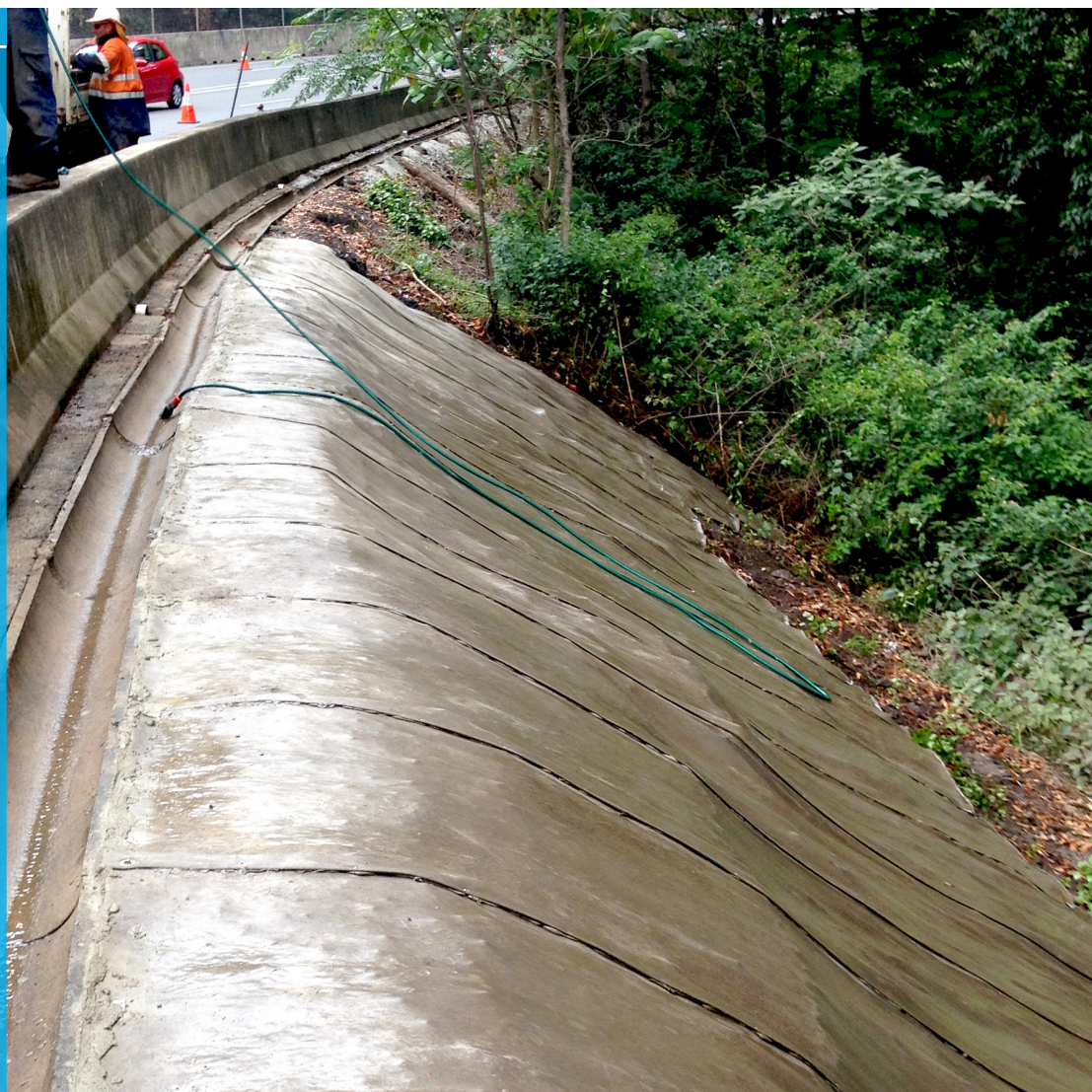
Section of slope immediately following hydration
