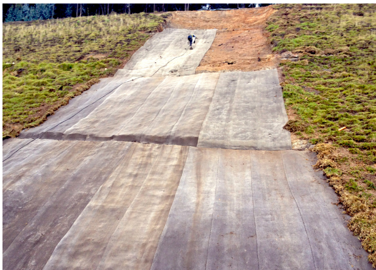
The CC was laid in vertical lengths, working from toe to crest
