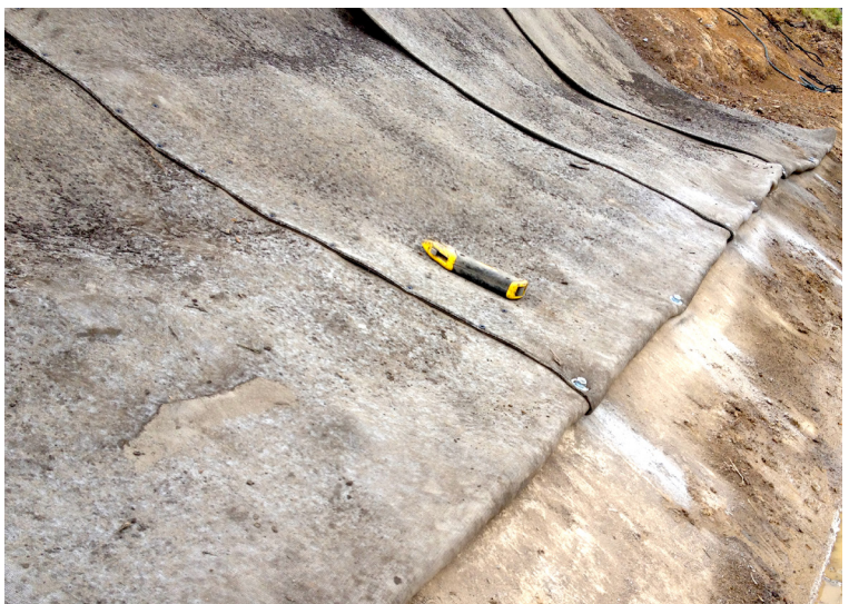
Hand tools were used to cut, fix and joint CC
