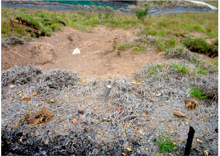
Bad weather and water runoff had caused severe erosion
