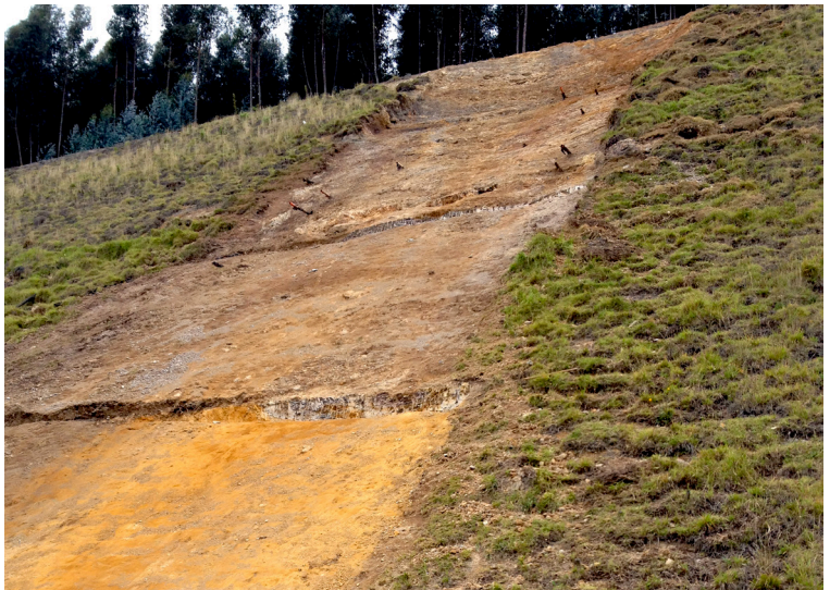
Ridges were created in the slope to dissipate water energy
