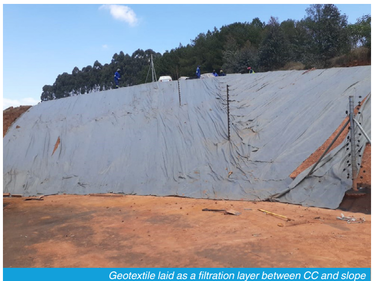
Geotextile laid as a filtration layer between CC and slope
