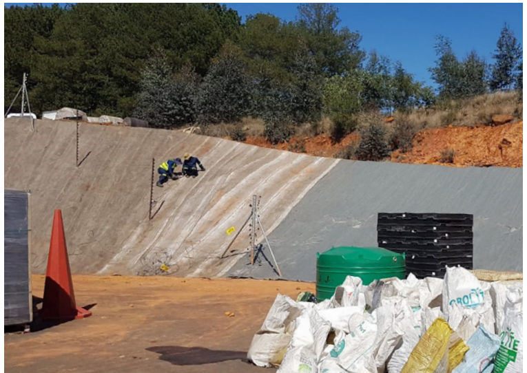
CC installed over geotextile barrier layer
