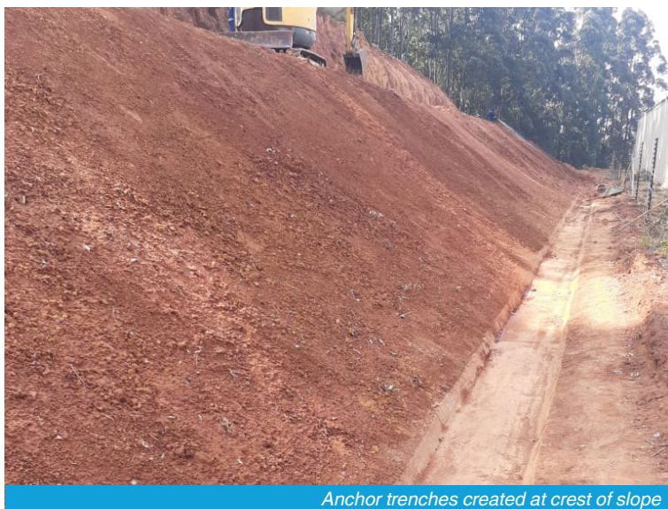
Anchor trenches created at crest of slope
