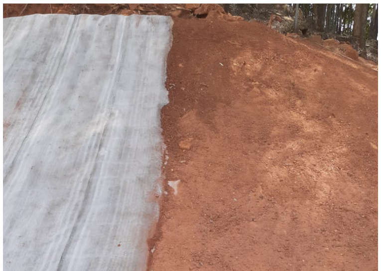
Open side edge buried in anchor trench
