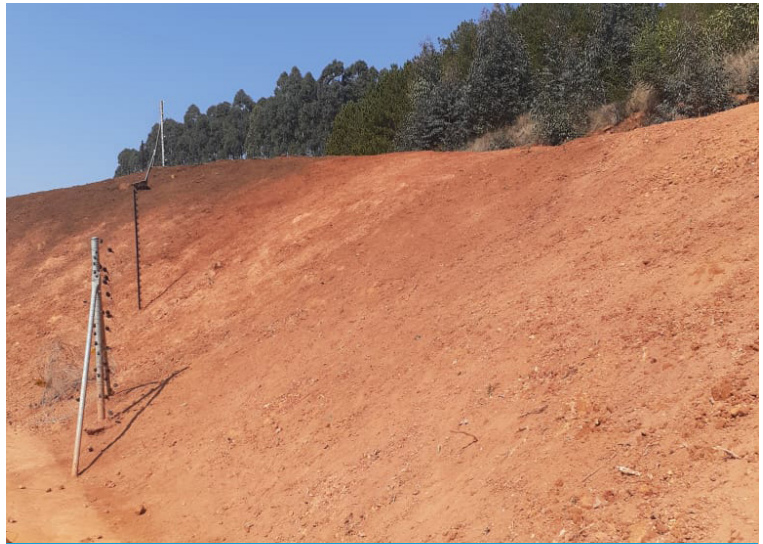
Rocks and boulders removed and slope face trimmed
