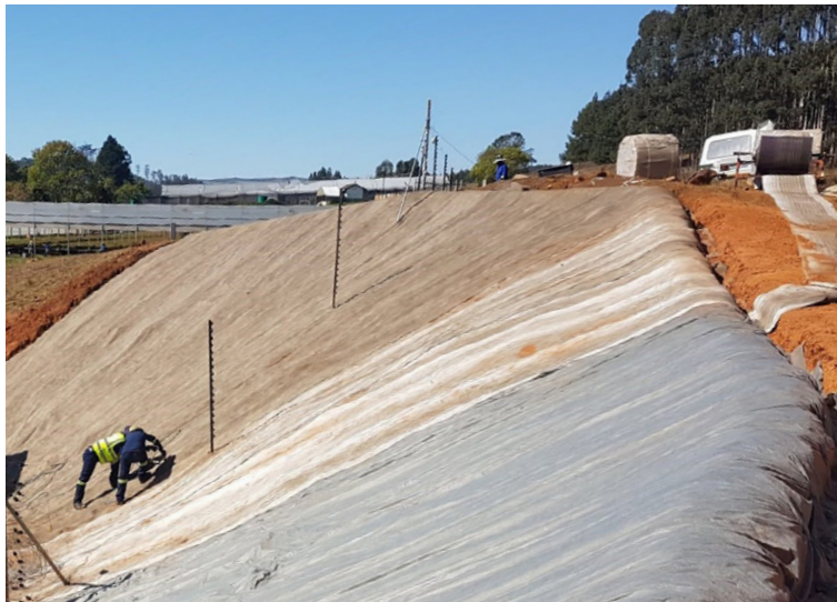
Bulk rolls dispensed at crest of slope and deployed vertically down slope face
