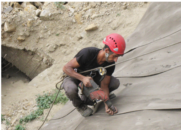
The CC was fixed with screws every 200mm
