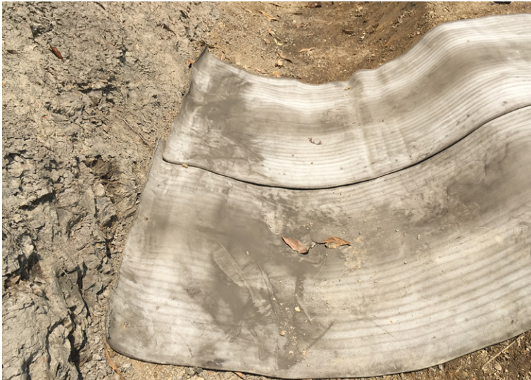
Leading edges of CC secured in crest anchor trench
