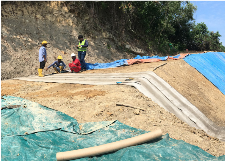
CC lengths laid vertically down slope face
