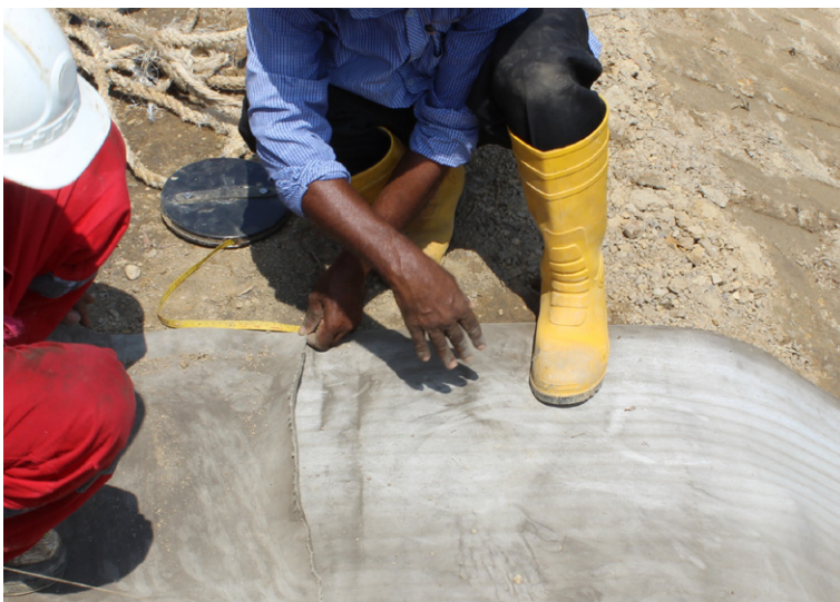
Additional lengths jointed along short edges
