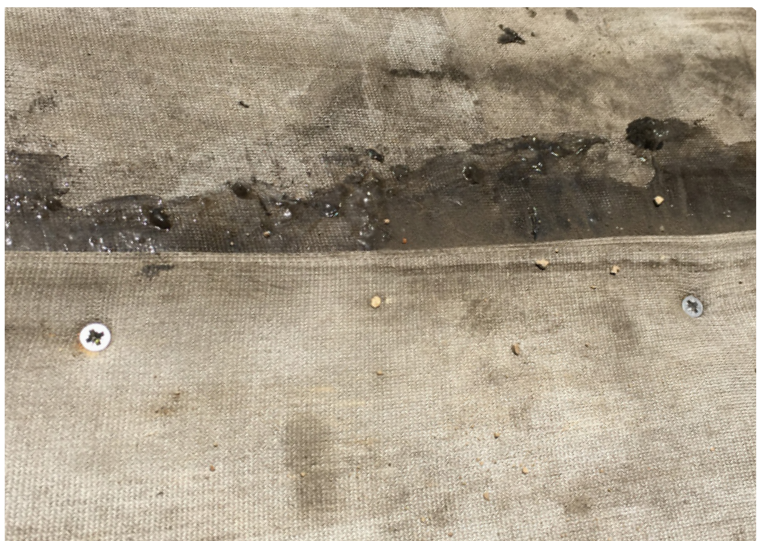
Stainless steel screws and sealant used for jointing overlaps
