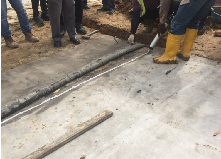
Sealant used to joint CC layers following hydration under overlap
