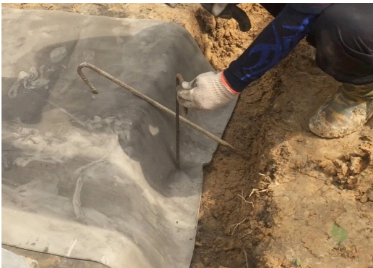
CC edges pinned within anchor trenches using ground pegs
