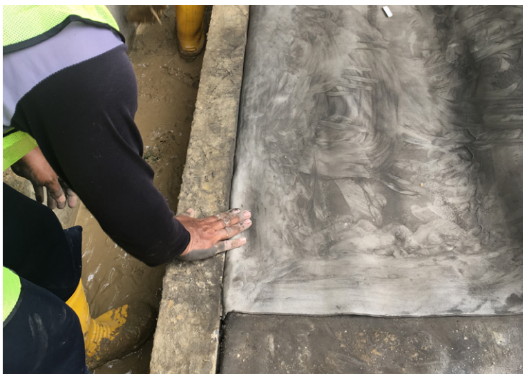
CC termination at toe
