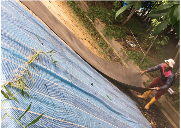
CC layers installed vertically
