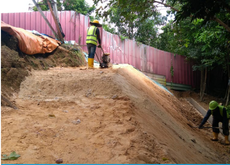
Compaction of slope following devegetation and grading
