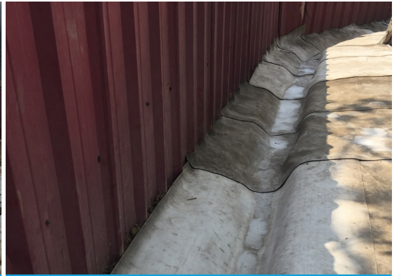
Additional drain at slope side
