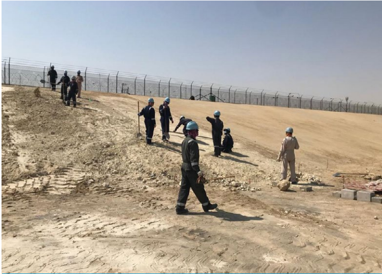
Slopes excavated and re-profiled
