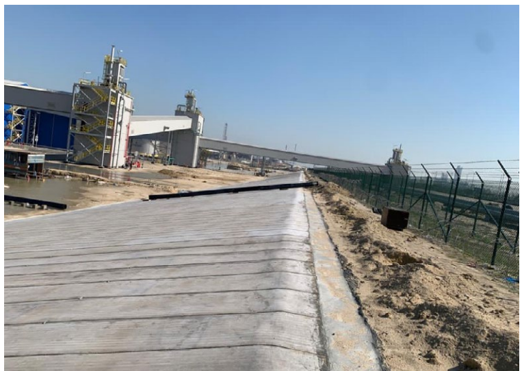
Anchor trench backfilled with concrete
