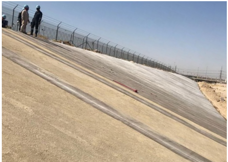
CC5™ laid vertically down the slope
