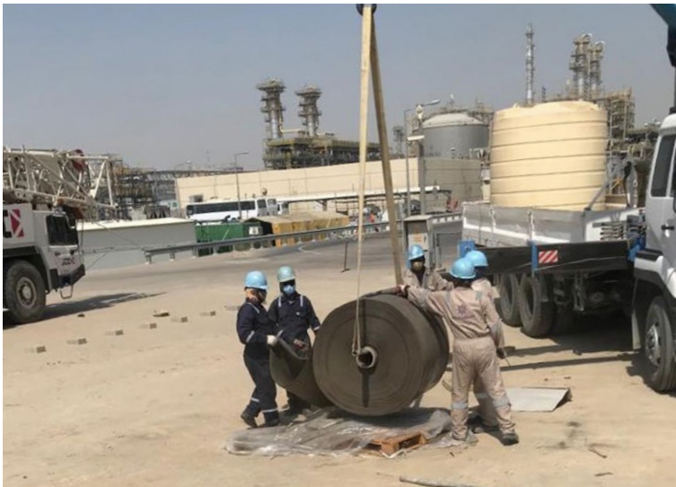
CC5™ Bulk Roll installed with the use of a spreader beam
