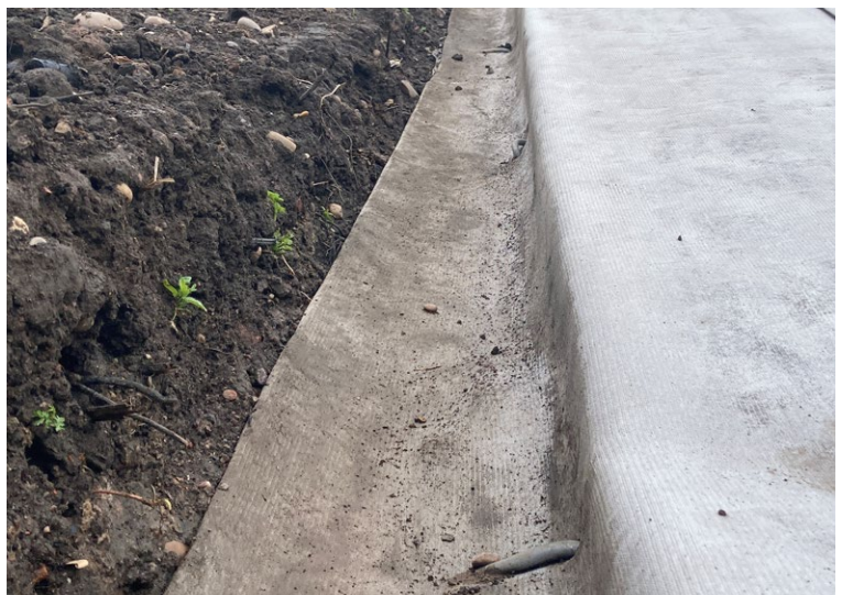
CC8™ secured in anchor trenches using stainless steel J-pegs
