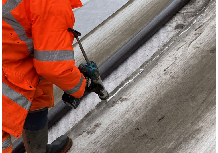
Adhesive sealant applied to reduce permeability of joints
