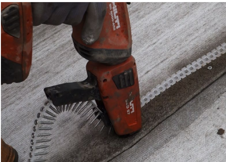
CC8™ layers secured using autofed screwdriver and stainless steel screws
