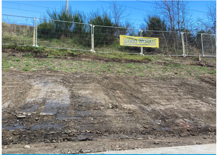
Slope reprofiled with vegetation removed
