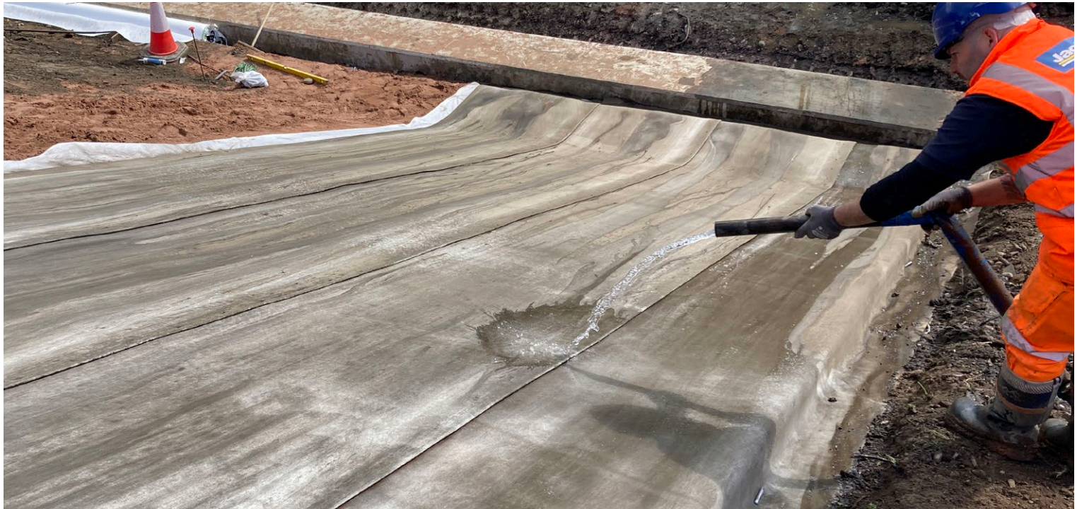
CC8™ material hydrated using a hose
