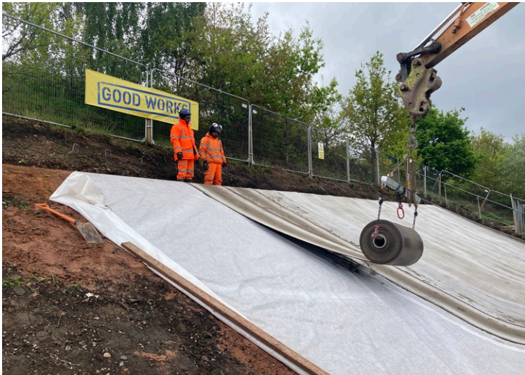
CC8™ Bulk Rolls laid vertically down the slope
