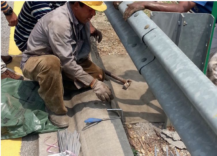
Fixing at crest with ground pegs
