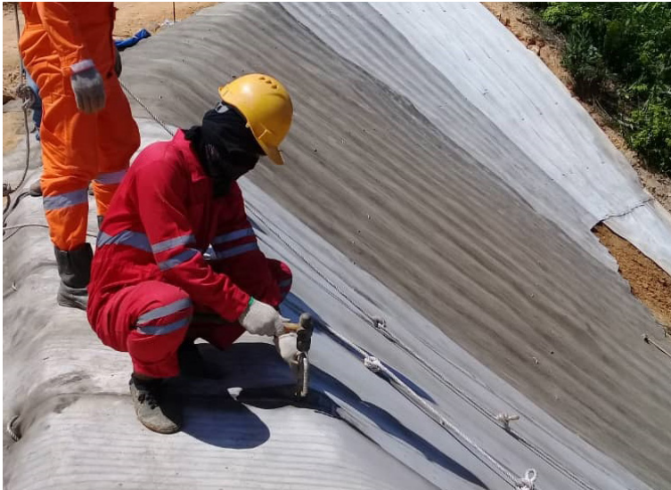
Using ground pegs to secure CC
