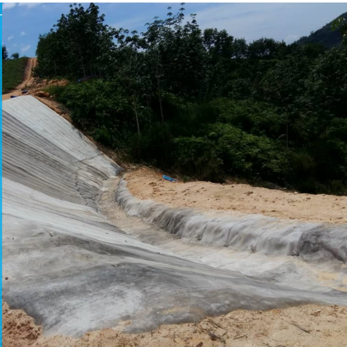
Completed slope protection installation
