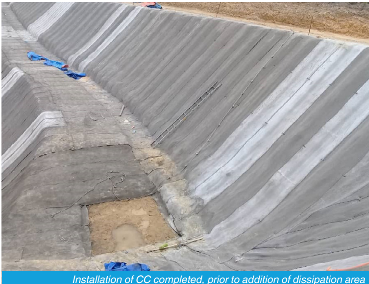
Using ground pegs to secure CC
