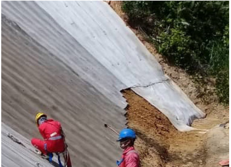
Fixing CC joints and example of sections overlapped in direction of water flow
