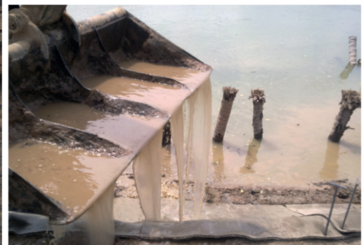
Hydration of the CC using plant site equipment
