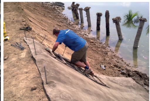
Pegging the pre-cut layers of CC to the substrate
