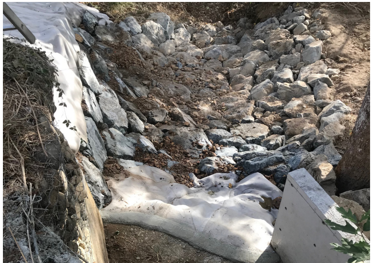
CC installed around drain outfall
