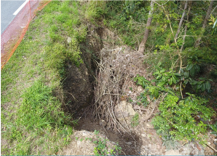
Section of slope affected by erosion and subsidence
