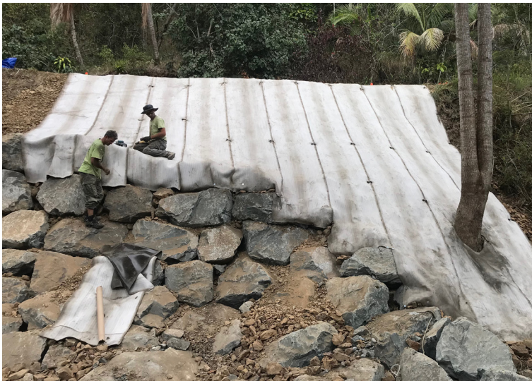
Cutting and fixing CC
