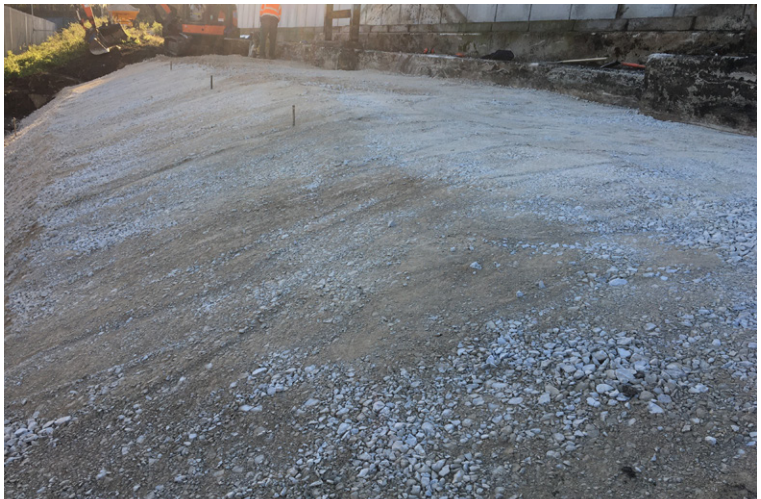
Type 2 hardcore was used to regrade the slope
