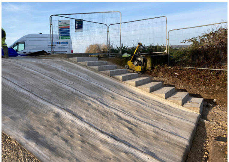
CC terminating into concrete stairs
