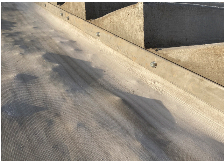
Termination at concrete stairway at one end of the slope
