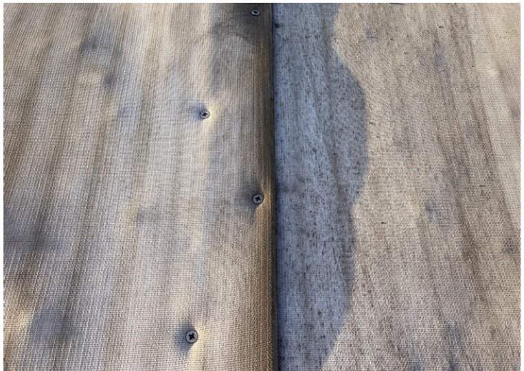
Screws were inserted in a zigzag formation to secure overlaps
