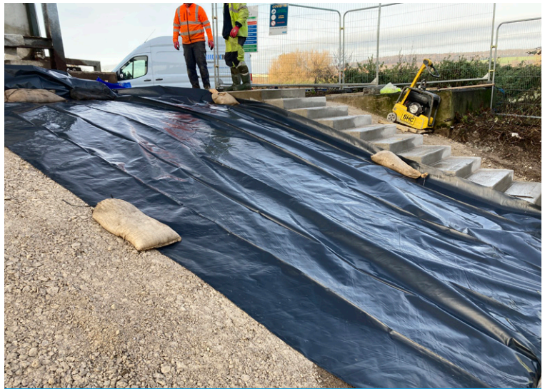
Plastic sheeting used to cover CC overnight to prevent freezing after hydration
