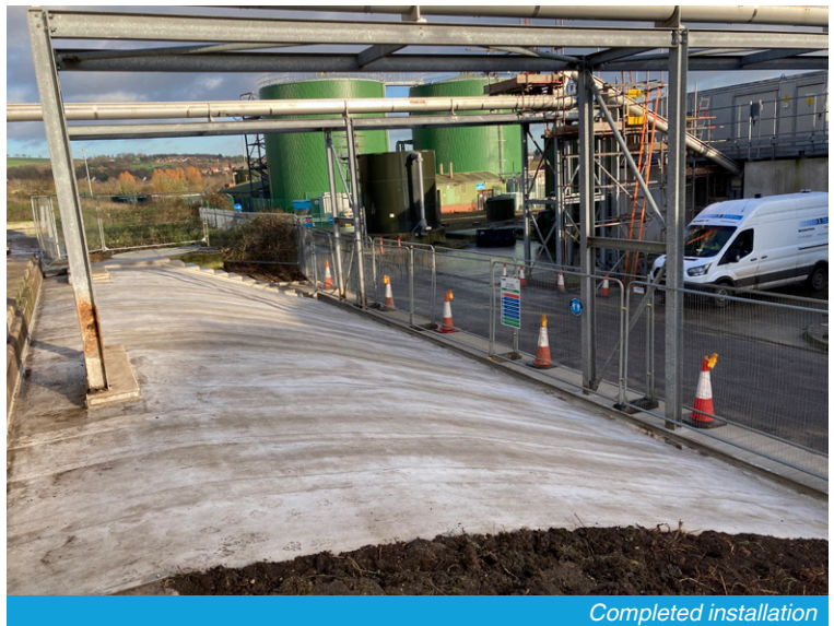
Plastic sheeting used to cover CC overnight to prevent freezing after hydration
