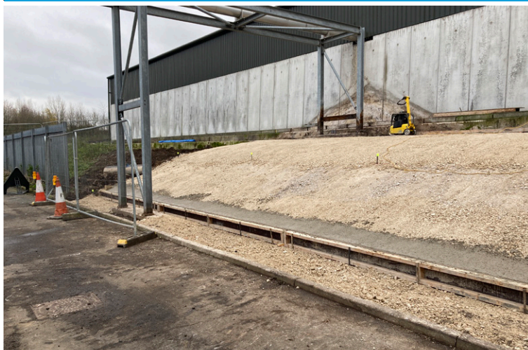
The hardcore was compacted to provide a uniform installation surface
