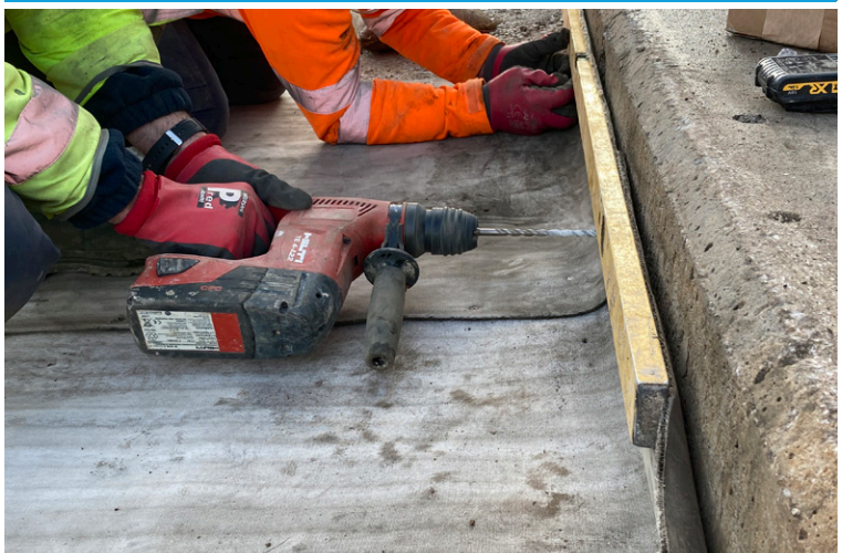
CC edges terminated against concrete upstand at the crest
