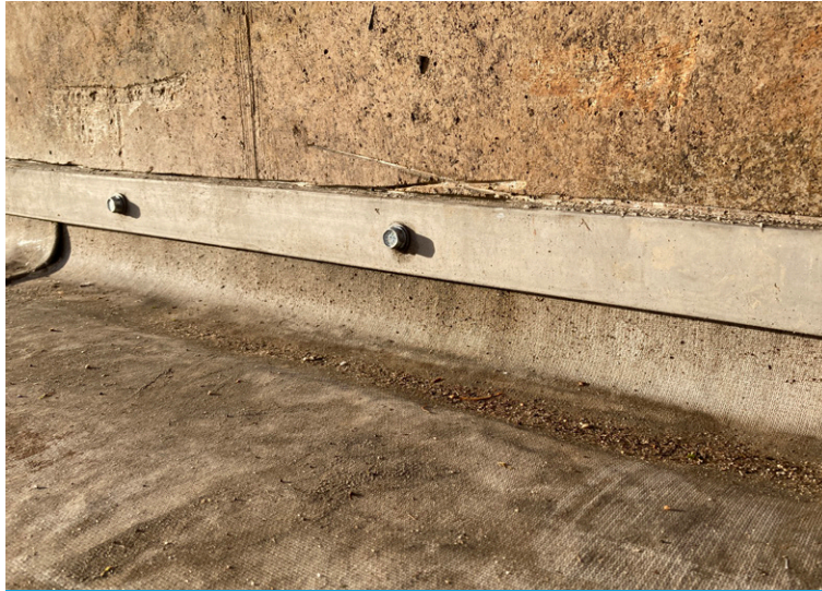
Stainless steel fixings and a termination bar were used at the crest
