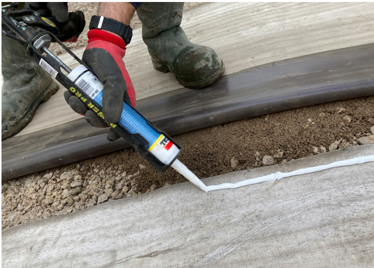
Adhesive sealant was applied to overlapping layers
