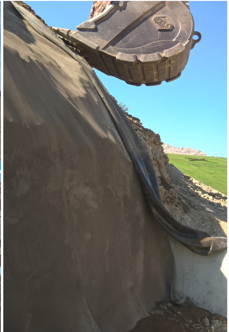
CC deployed using excavator
