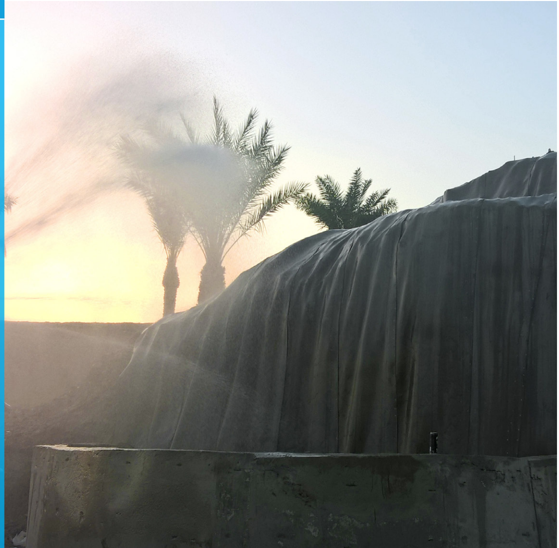
CC lined waterfall slope and water collection pool being hydrated
