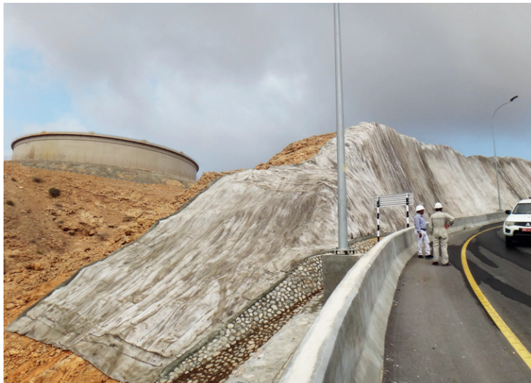
The end of the slope was covered using longitudinal and transverse layers
