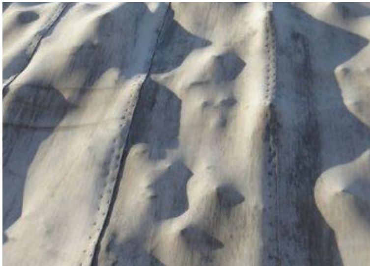
Overlapping layers of CC were secured with adhesive sealant and screws
