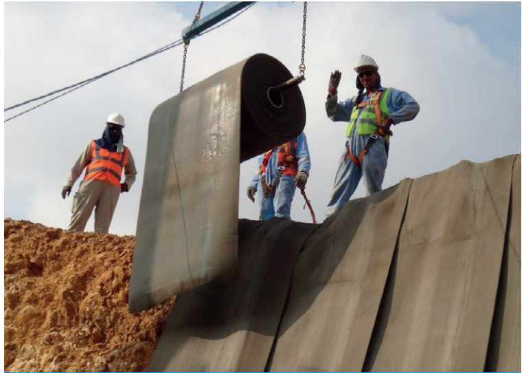
The CC was suspended from a spreader beam and excavator for unrolling
