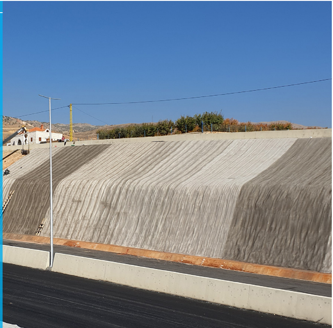
CC Slope Protection installation alongside the Pan Arab Highway in Lebanon
