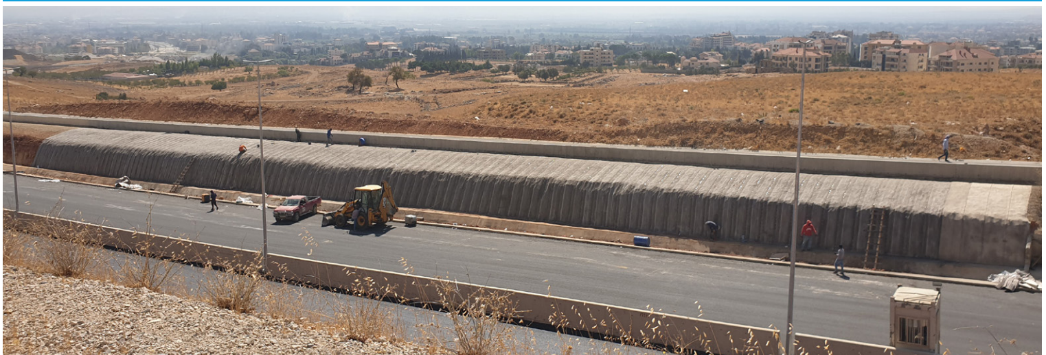
A total of 9600m 2 of CC5™ were installed as a slope protection solution alongside a stretch of the Pan Arab highway in Lebanon
