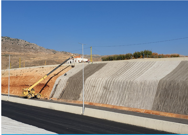
First section of slope protection installation in progress
