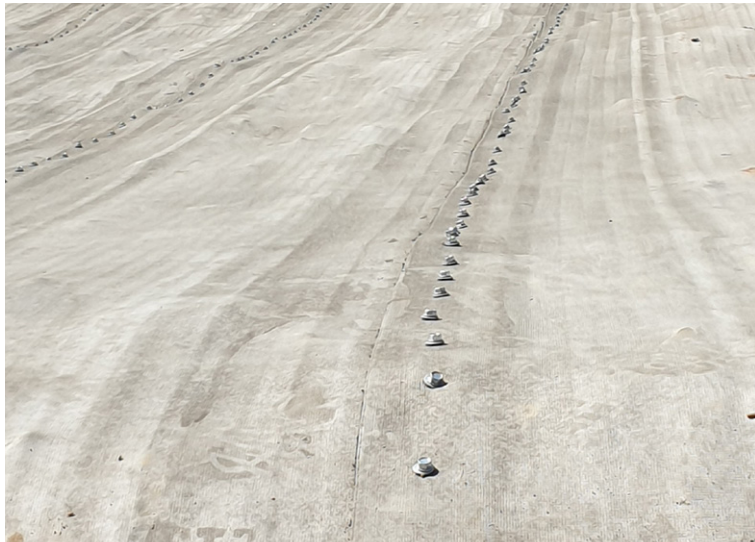
Overlapping layers thermally bonded and reinforced with anchor bolts
