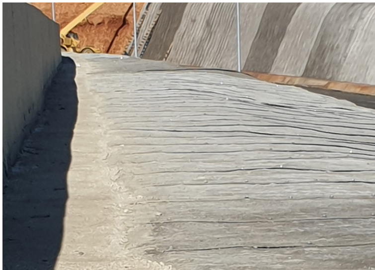
Concrete backfilled anchor trenches for ingress prevention & neat termination
