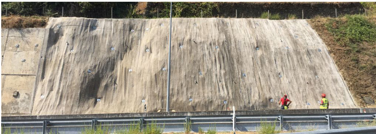
The completed installation of slope 1 - 320m 2
