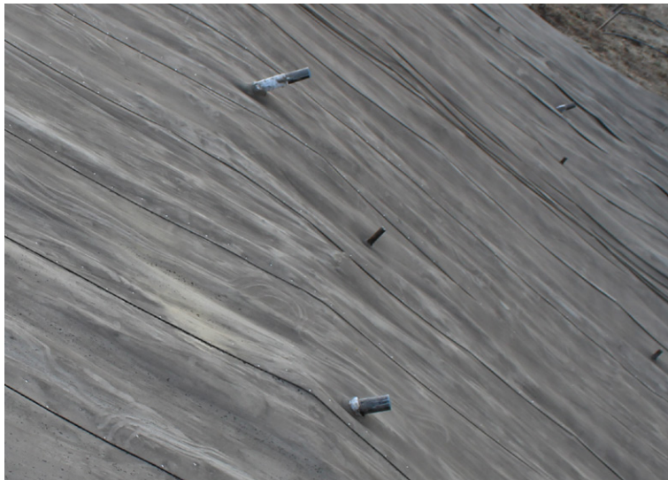
Holes were cut for any protruding elements
