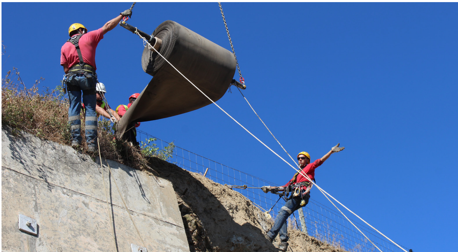
The Concrete Canvas was attached to the existing concrete infrastructure on the one side with masonry screws
