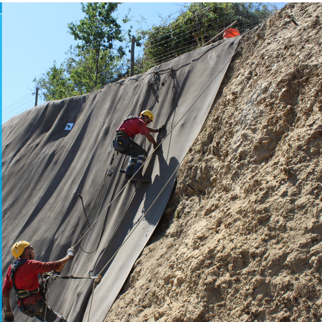
Each bulk roll was positioned at the top of the slope and unrolled downwards
