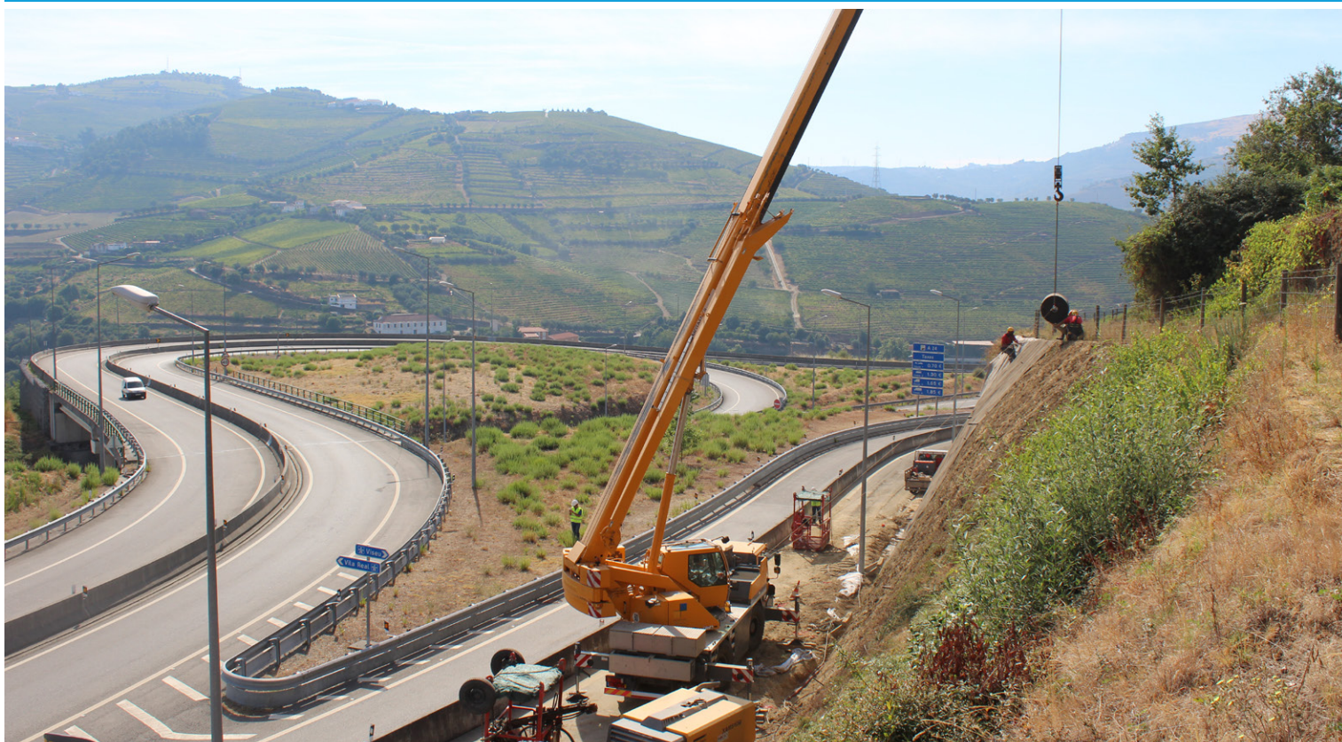
The CC was mounted onto a spreader beam and hung from a truck crane stationed at the base of each slope
