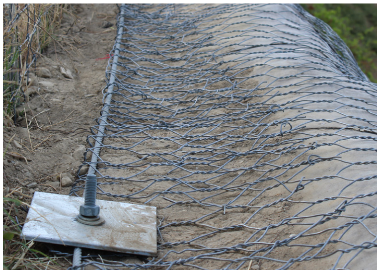
Face plates were used to anchor a wire mesh in place
