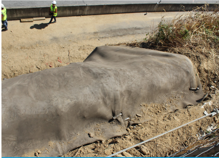
380mm ground pegs were inserted every 1m
