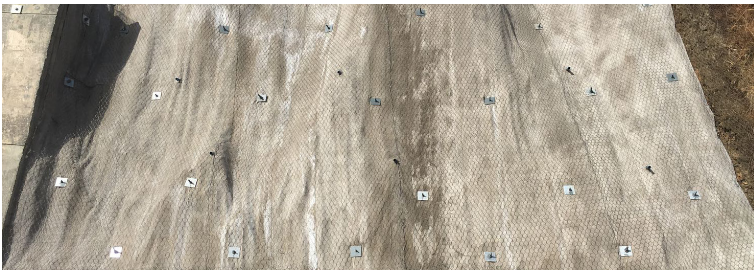
In total, 480m 2 of CC5™ (Slope 1 - 320m 2 & Slope 2 - 160m 2 ) was installed by 4 people in under 3 (8hr) days on both slopes with restricted access
